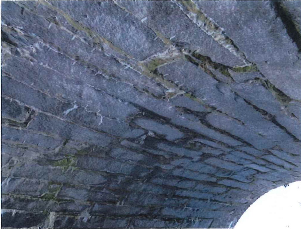
Photo 13: Typical condition of the underside of the arch.
