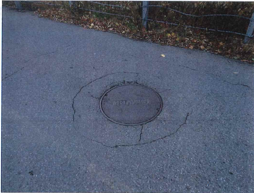
Photo 5: Manhole in the Southbound lane of the North approach.
