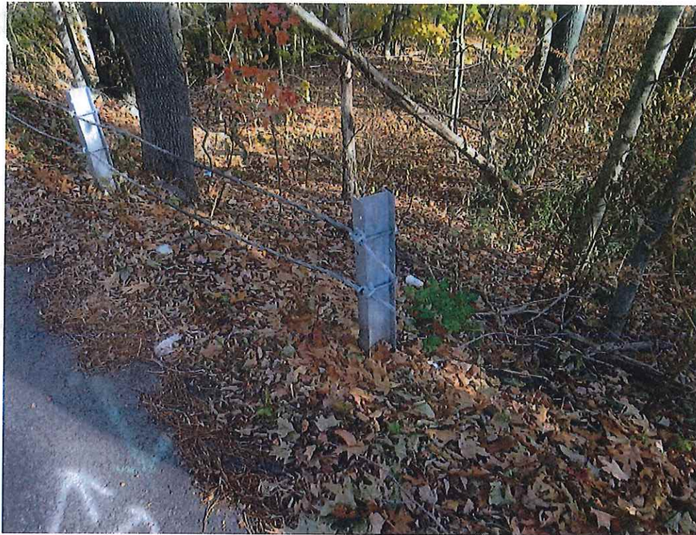
Photo 15: Southeast approach guardrail end.
