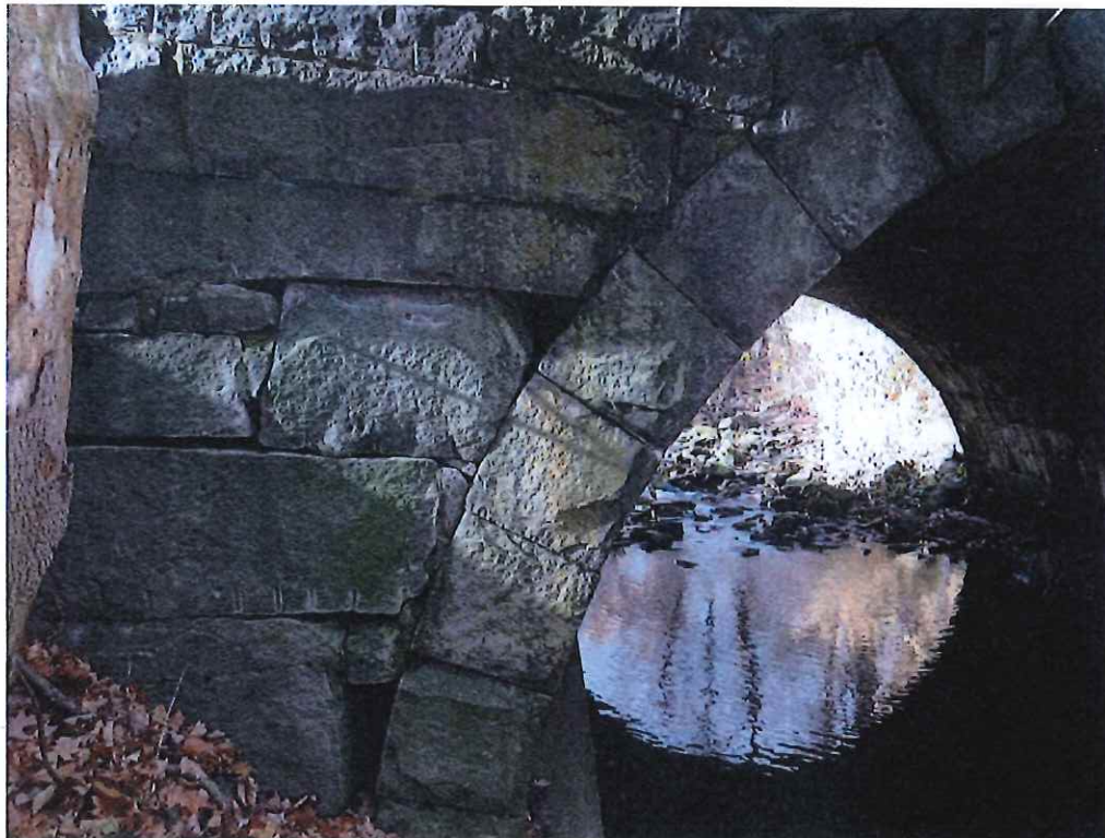
Photo 6: East spandrel wall along the South end of the arch ring.
