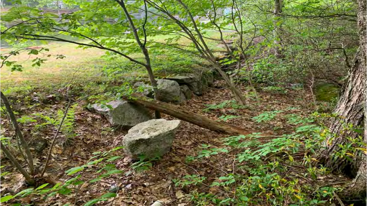
Photo 9: Right downstream face from the right abutment – Missing cap stones along the top of the wall in multiple locations. Heavy vegetation was observed within 20 feet of the toe.
