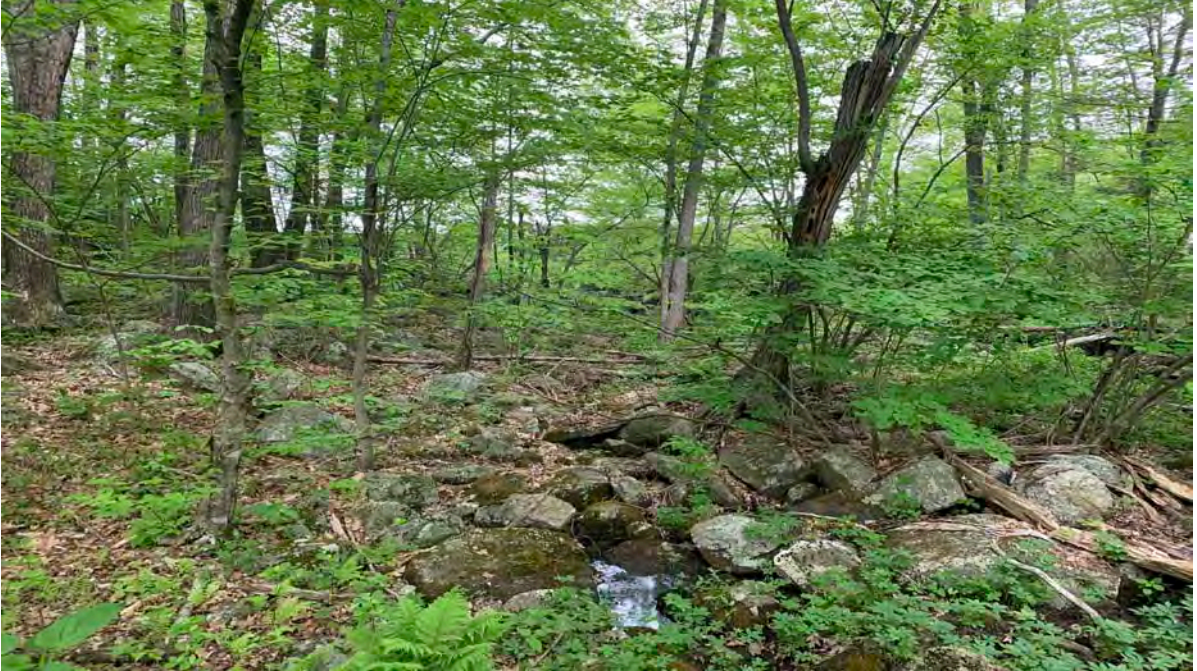
Photo 17: Downstream area along the channel looking back at the dam. The area is heavily vegetated with many trees within 20 feet of the dam toe.
