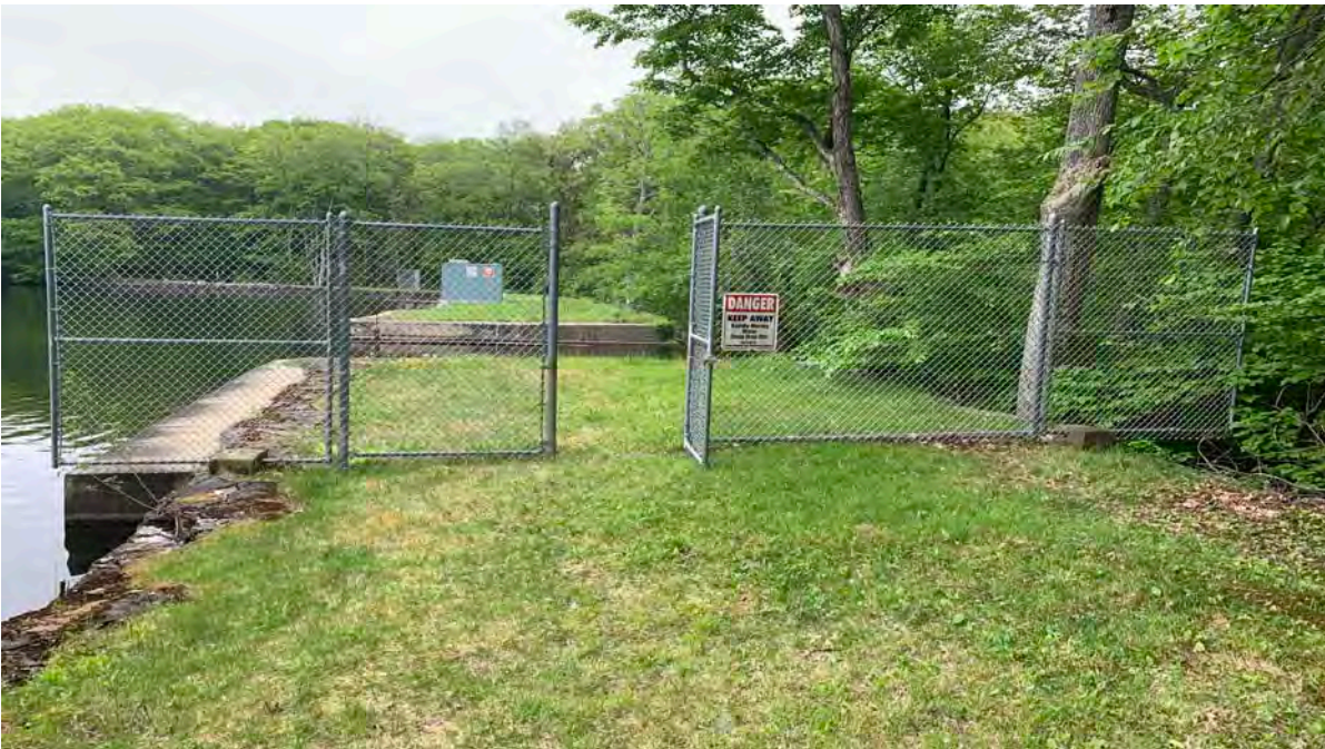
Photo 6: Right crest from the right abutment – There was some thin vegetation along the crest. Note the gate located across the crest.
