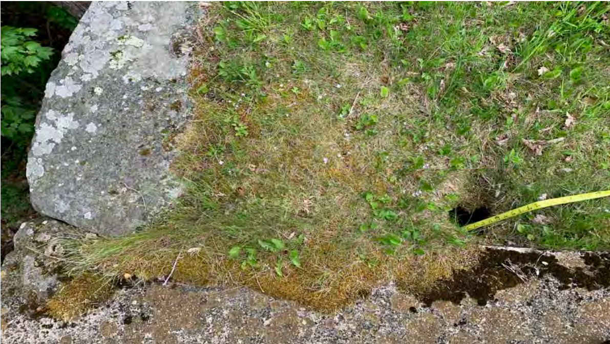
Photo 8: Void in right crest adjacent to the right spillway training wall.
