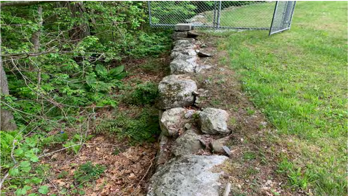
Photo 10: Left downstream face from the left abutment – Missing cap stones along the top of the wall in multiple locations. Heavy vegetation was observed within 20 feet of the toe.
