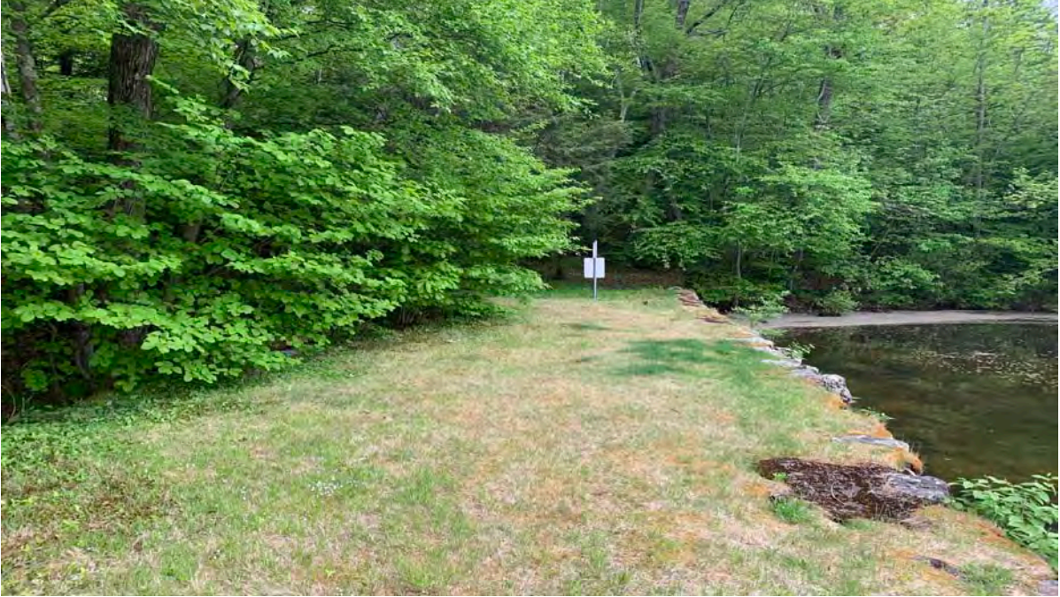
Photo 1: Right abutment from dam crest – Vegetation within 20 feet of the contact mainly on the upstream and downstream sides.
