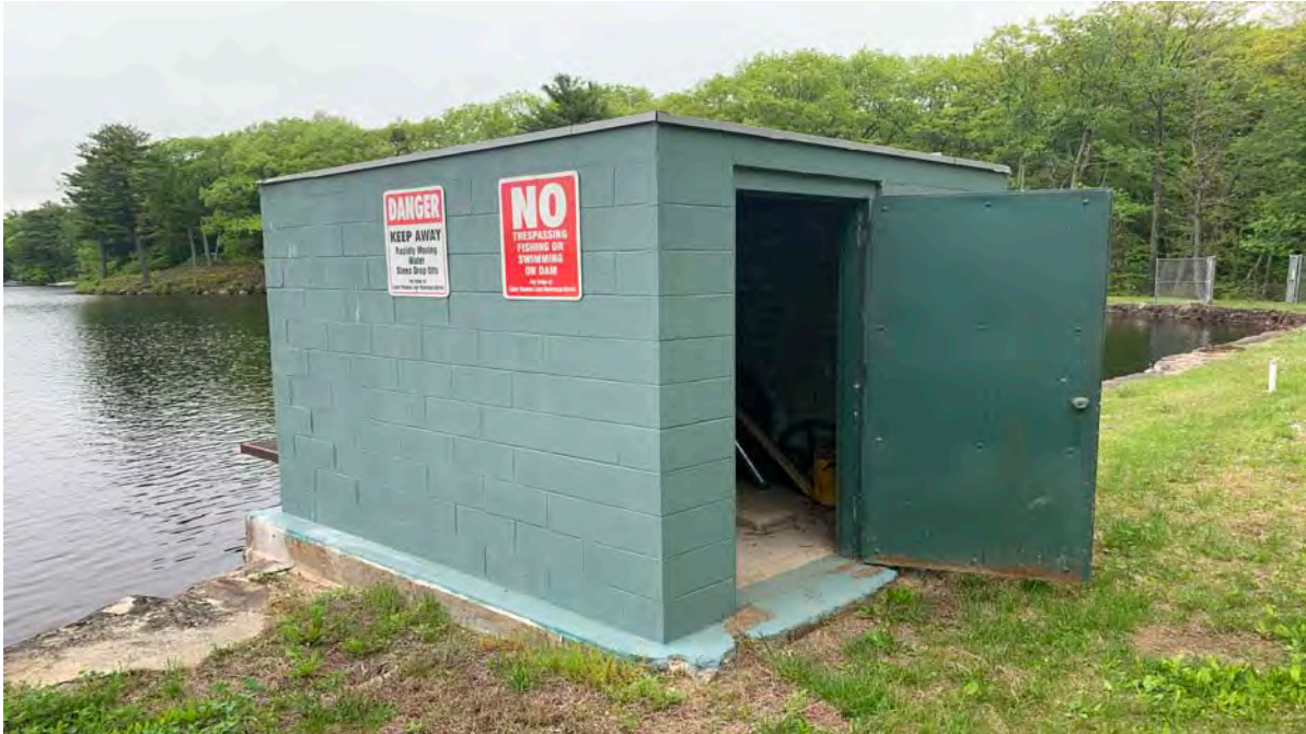
Photo 15: Gate house – The gate house was recently rebuilt but no longer serves a function other than storage. Access to the controls is through this building out onto a cantilever platform.
