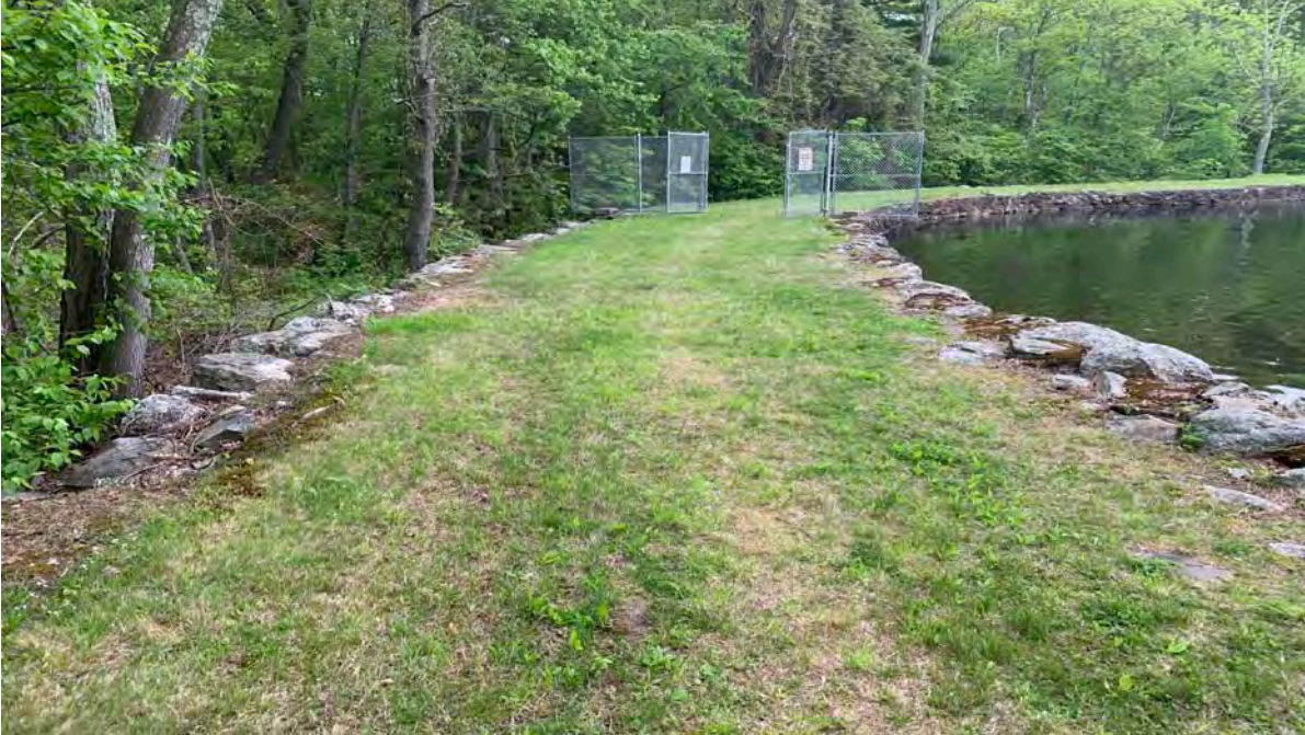
Photo 7: Left crest from the left abutment – There was some thin vegetation along the crest as well as some shallow tire rutting. Note the gate located across the crest.
