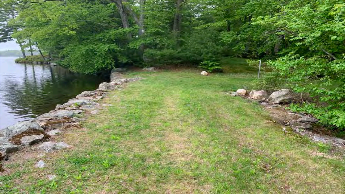
Photo 3: Left abutment from the crest – Minor thin areas of vegetation and shallow tire rutting.
