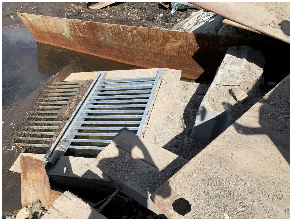
Photo 2: Overview of the Low-Level Outlet Intake.
