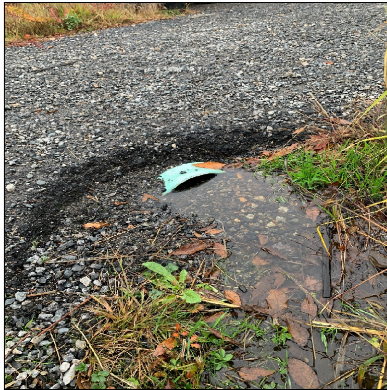
Photo 2: Existing 10-inch PVC pipe to the west of the parking lot.
