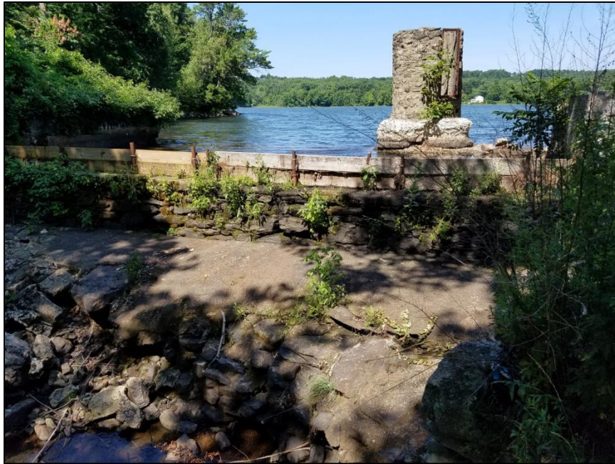
Photo 9: Overview of spillway from downstream
