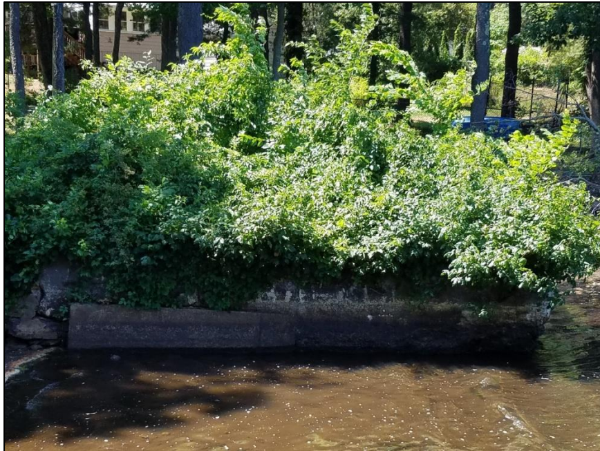
Photo 5: Overview of dam crest facing right abutment
