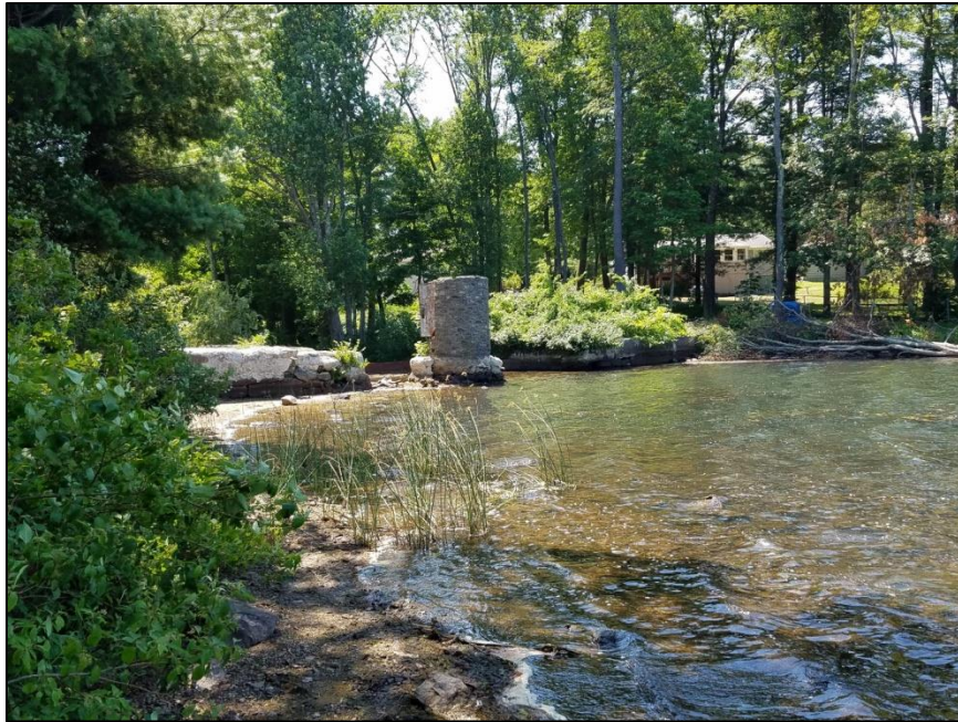
Photo 1: Overview of dam from upstream
