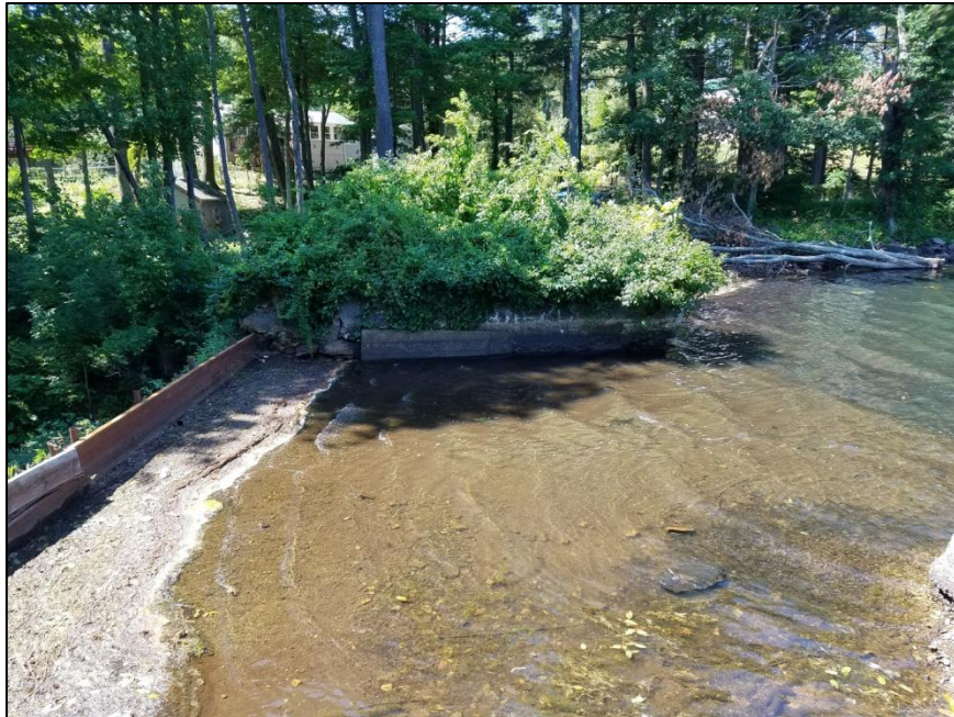
Photo 11: Overview of right training wall
