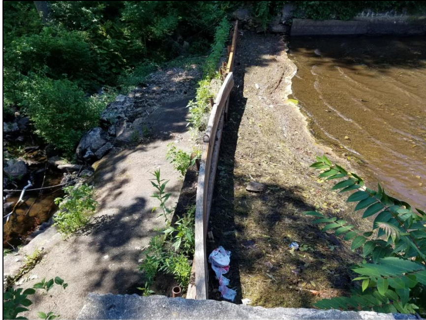
Photo 13: Overview of spillway from left training wall
