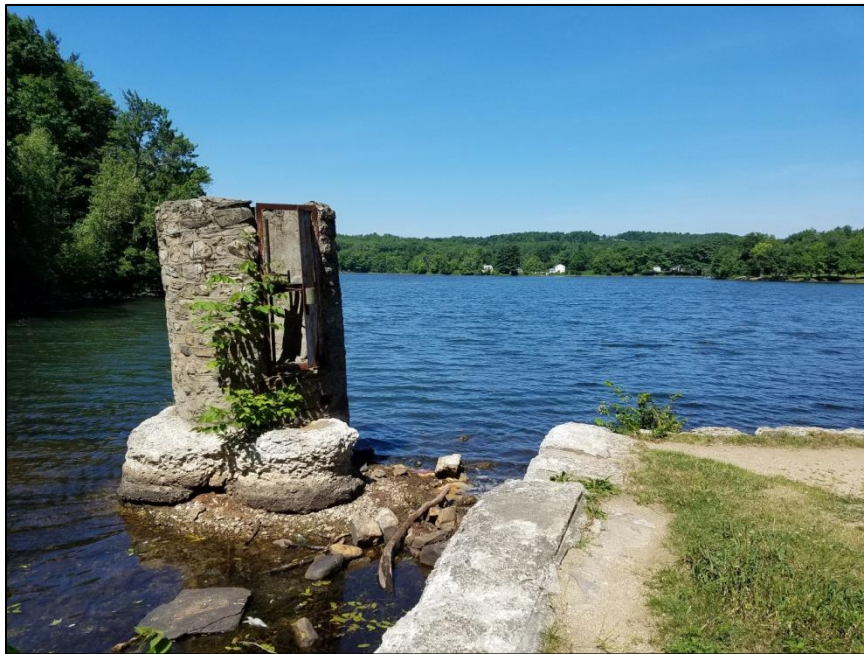
Photo 24: Overview of impoundment (Waite Pond)
