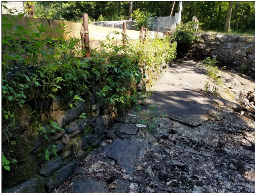
Photo 10: Overview of spillway from downstream
