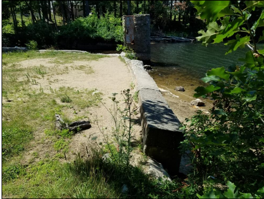
Photo 3: Overview of upstream face from left abutment
