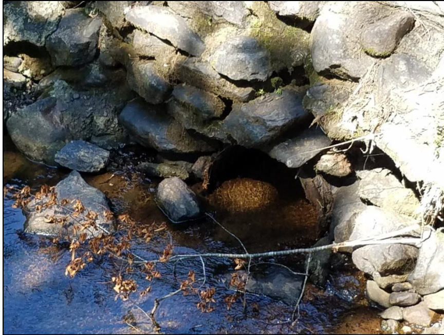
Photo 23: Low-level outlet pipe
