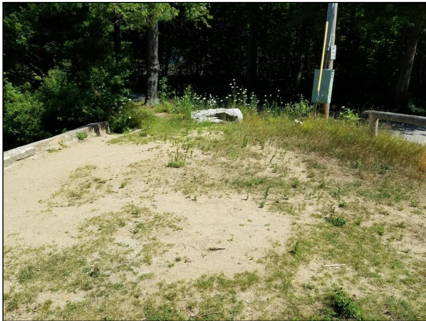
Photo 4: Overview of dam crest facing left abutment
