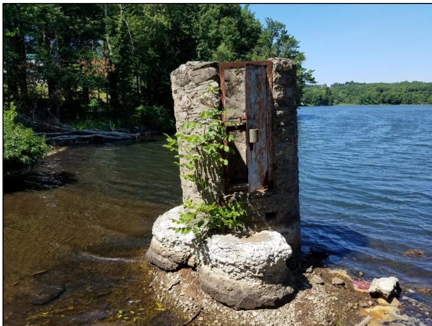
Photo 16: Overview of gatehouse exterior
