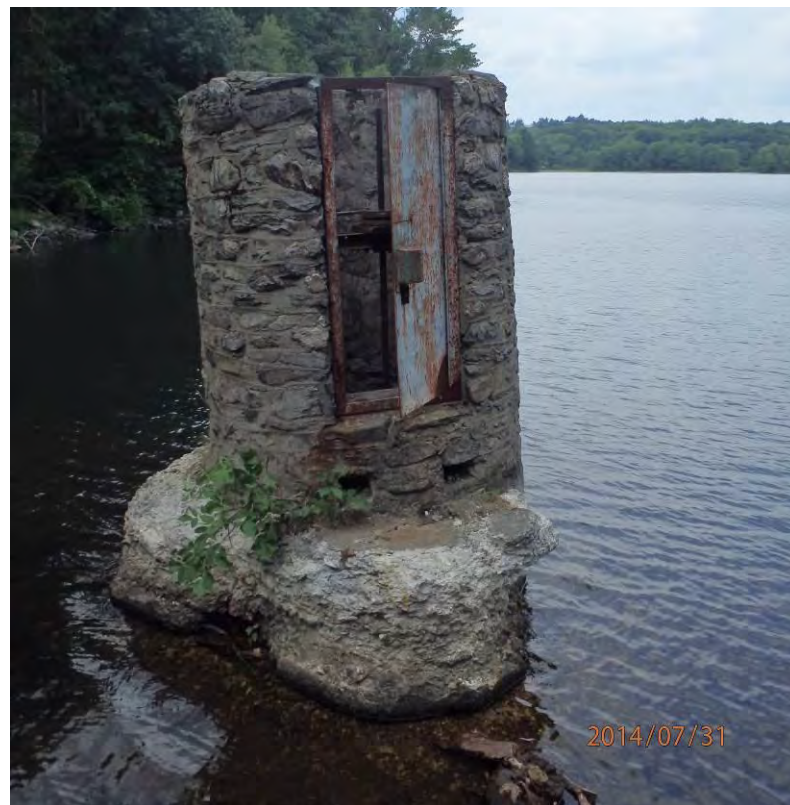
Photo 12: Overview of gatehouse exterior
