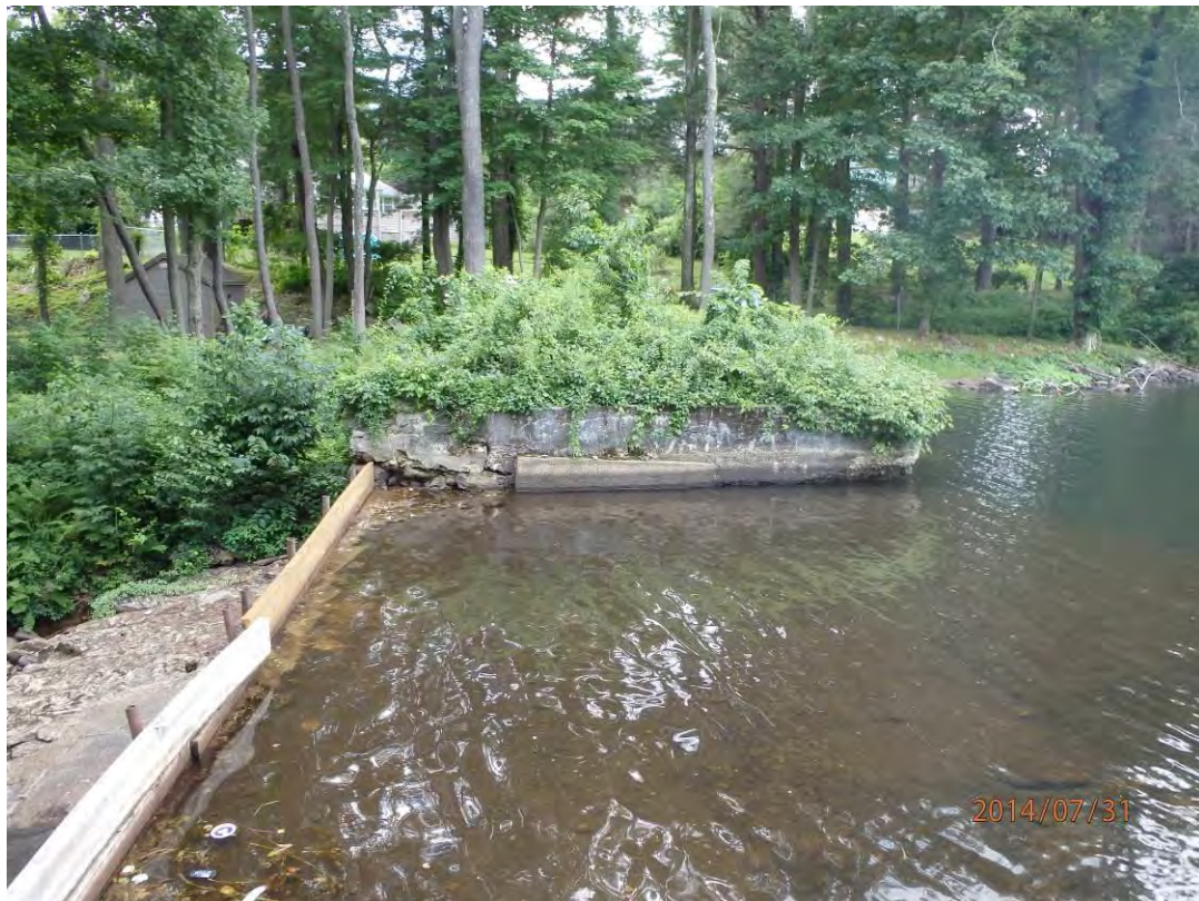
Photo 8: Overview of right training wall
