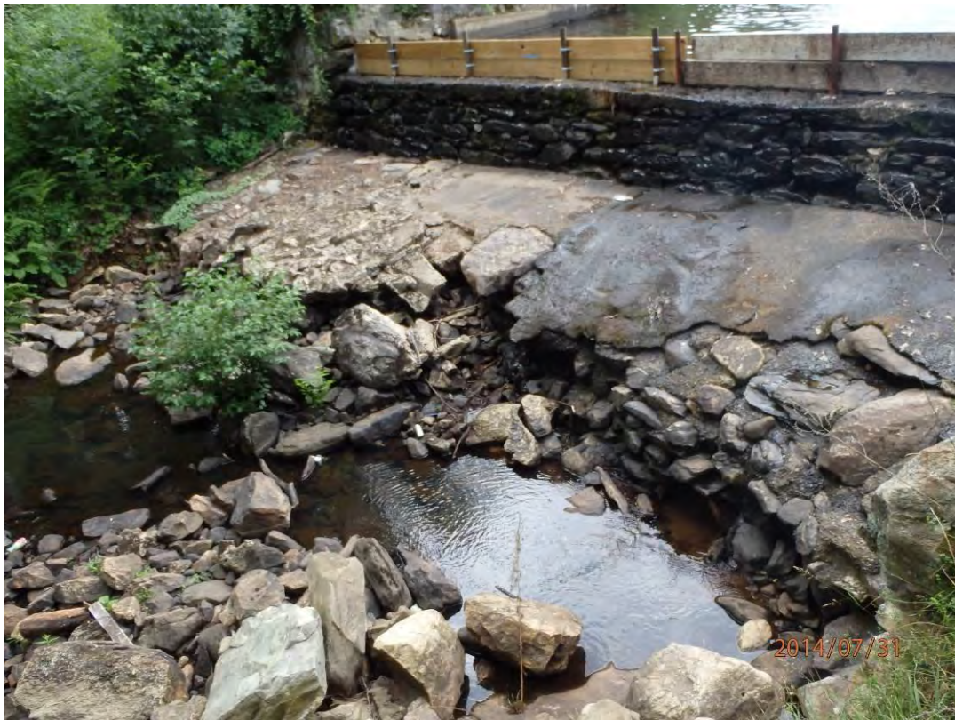
Photo 10: Overview of stilling basin & low-level outlet discharge location
