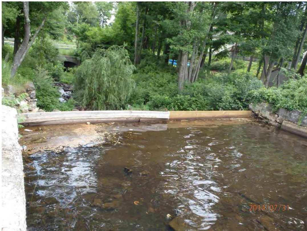
Photo 6: Overview of spillway from upstream
