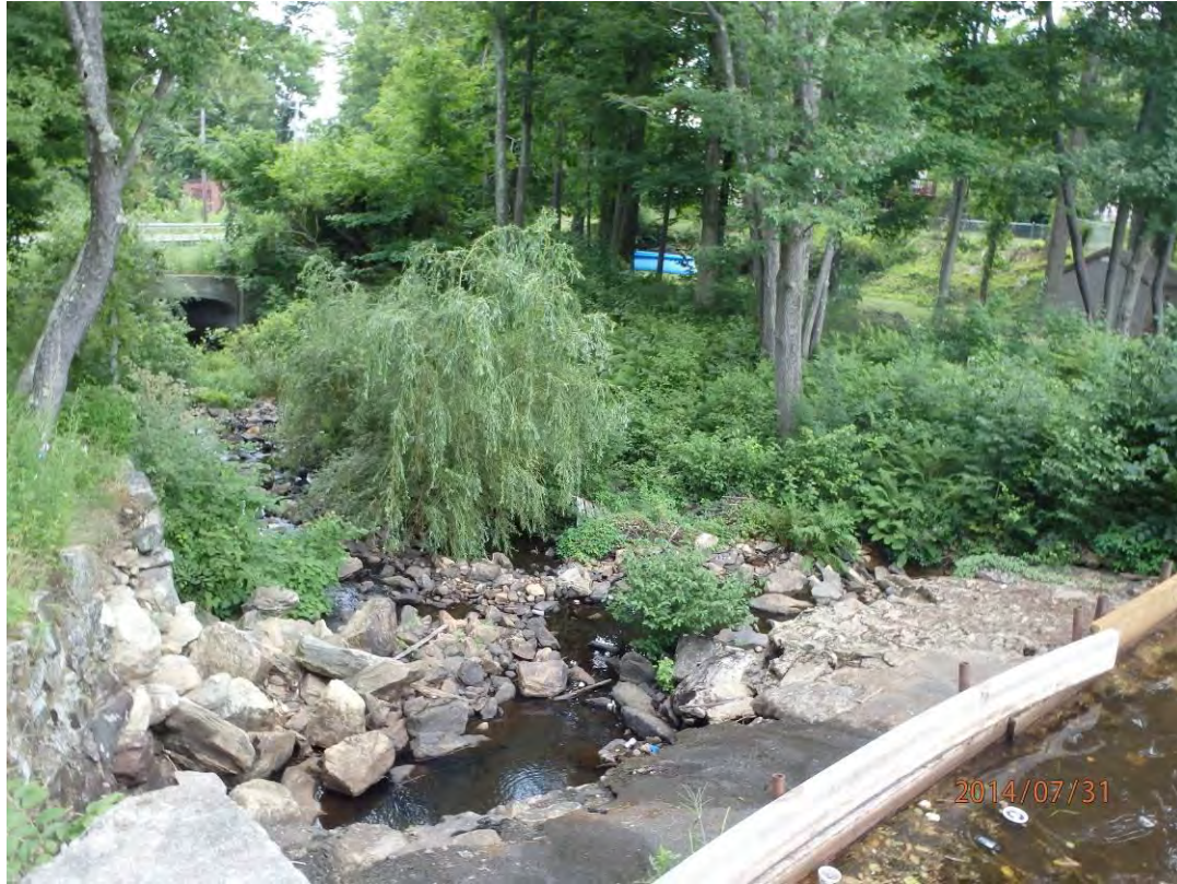
Photo 11: Overview of downstream channel
