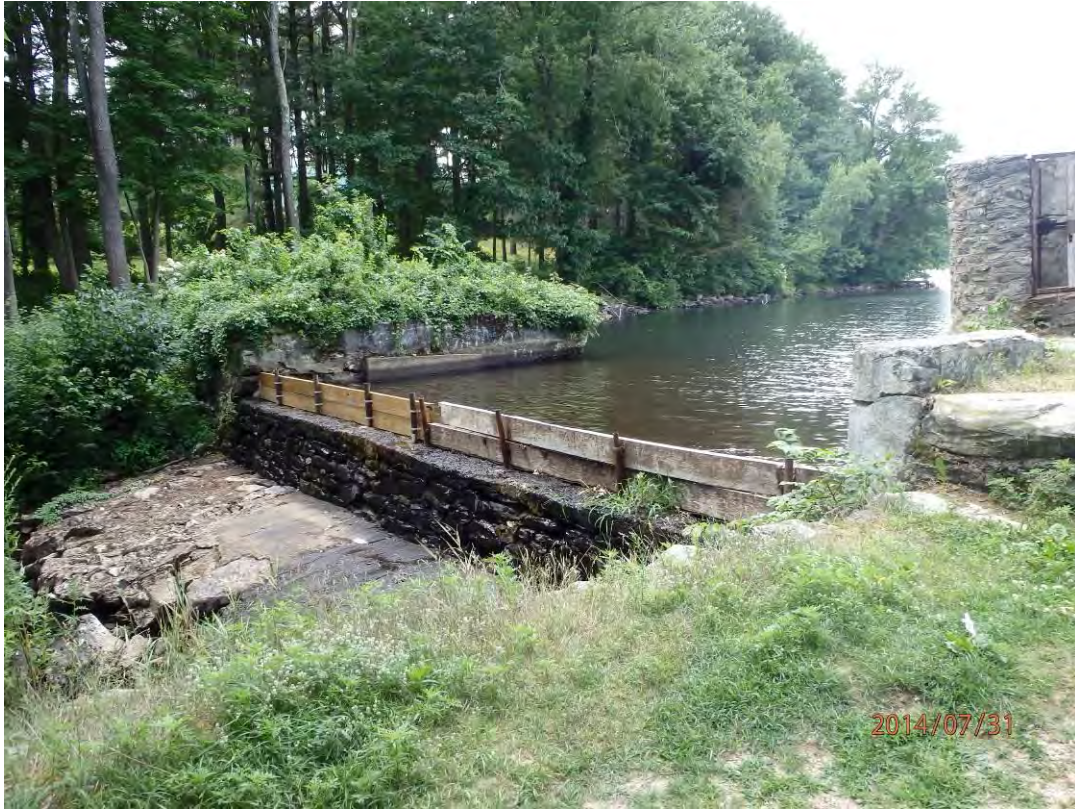
Photo 9: Overview of weir
