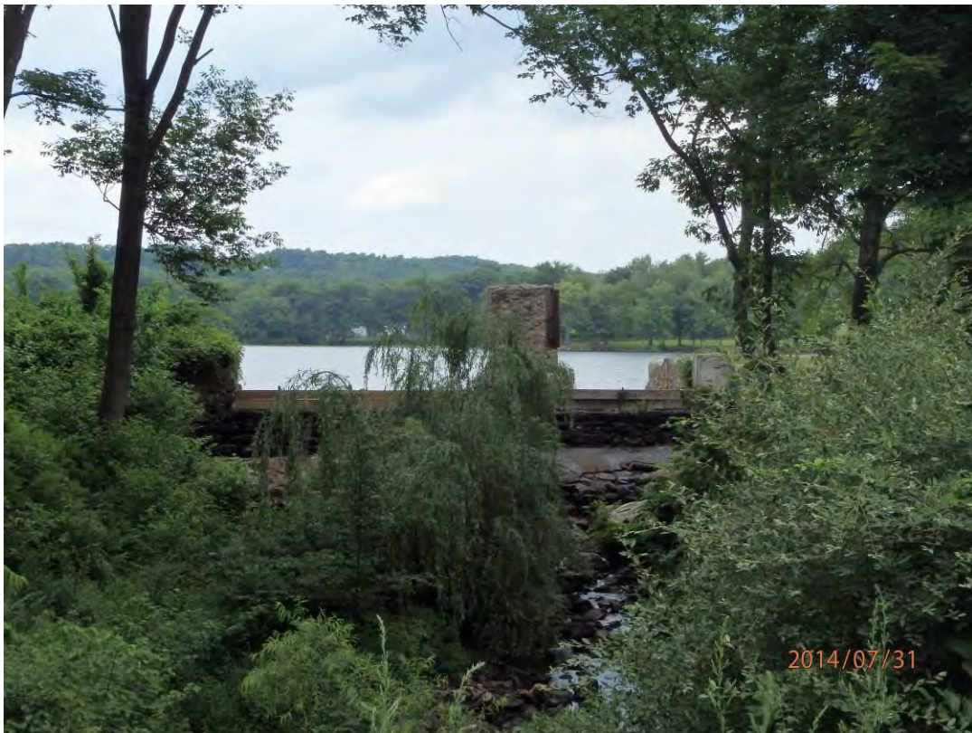
Photo 2: Overview of dam from downstream
