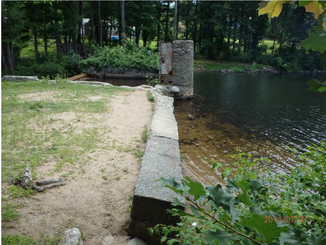
Photo 3: Overview of upstream face from left abutment
