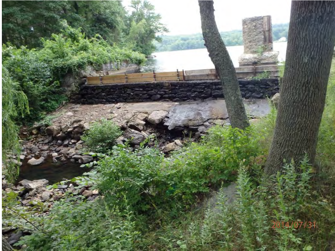
Photo 7: Overview of spillway from downstream (tailrace or channel area)
