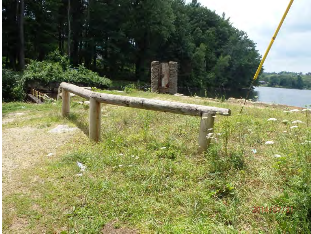
Photo 5: Overview of downstream face from left abutment
