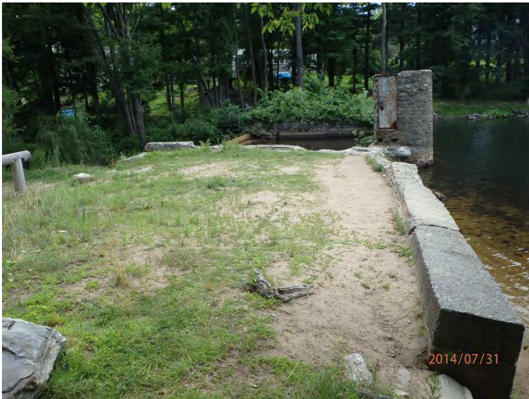
Photo 4: Overview of dam crest from left abutment
