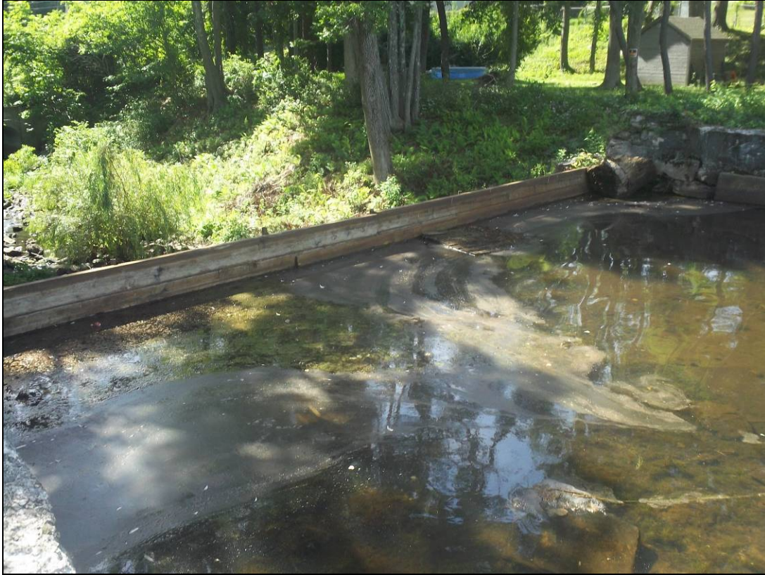
Photo 9: Overview of spillway from upstream
