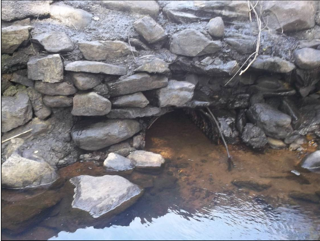
Photo 18: Low level outlet – 24” CMP
