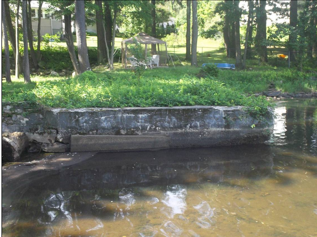
Photo 11: Overview of right training wall
