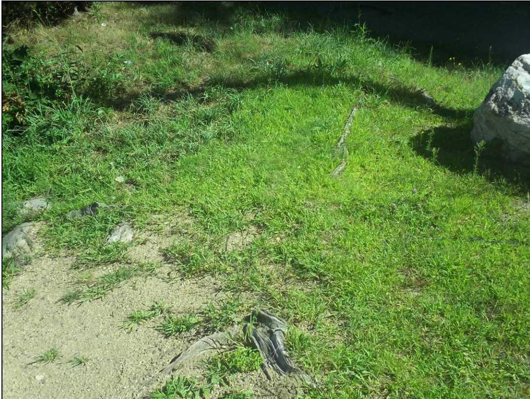
Photo 20: Areas of specific deficiencies-tree roots, sparse vegetative cover
