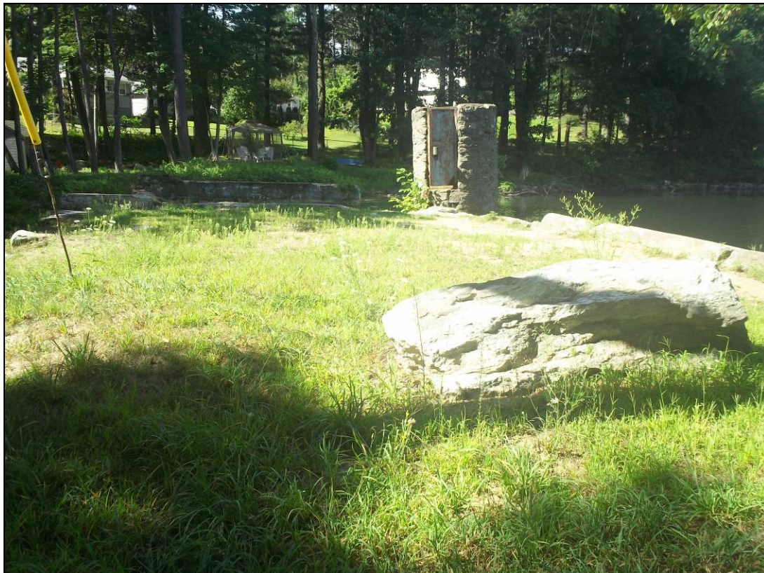
Photo 6: Overview of dam crest from left abutment
