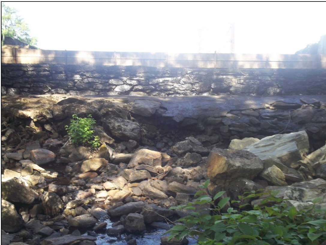
Photo 10: Overview of spillway from downstream (tailrace or channel area)
