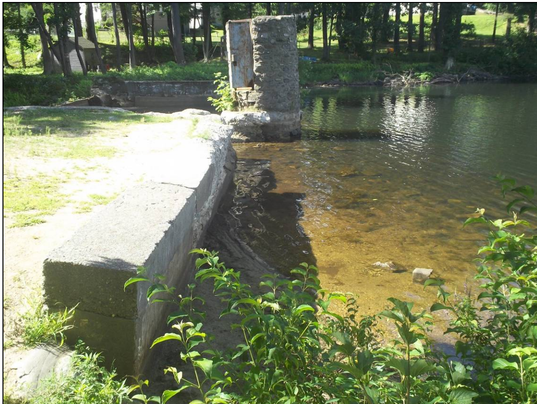
Photo 4: Overview of upstream face from left abutment
