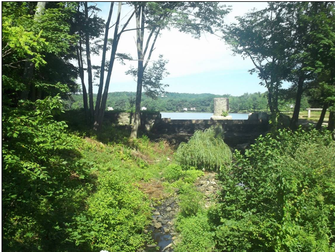
Photo 2: Overview of dam from downstream
