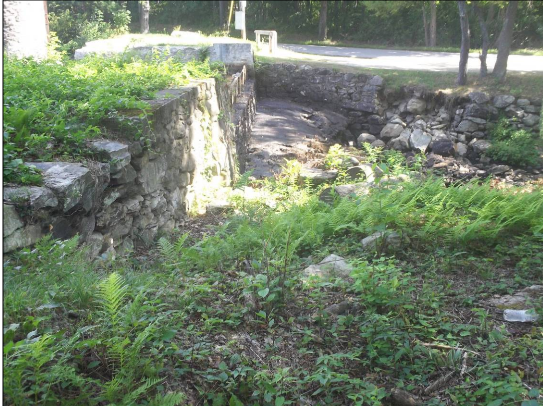
Photo 7: Overview of downstream face from right abutment
