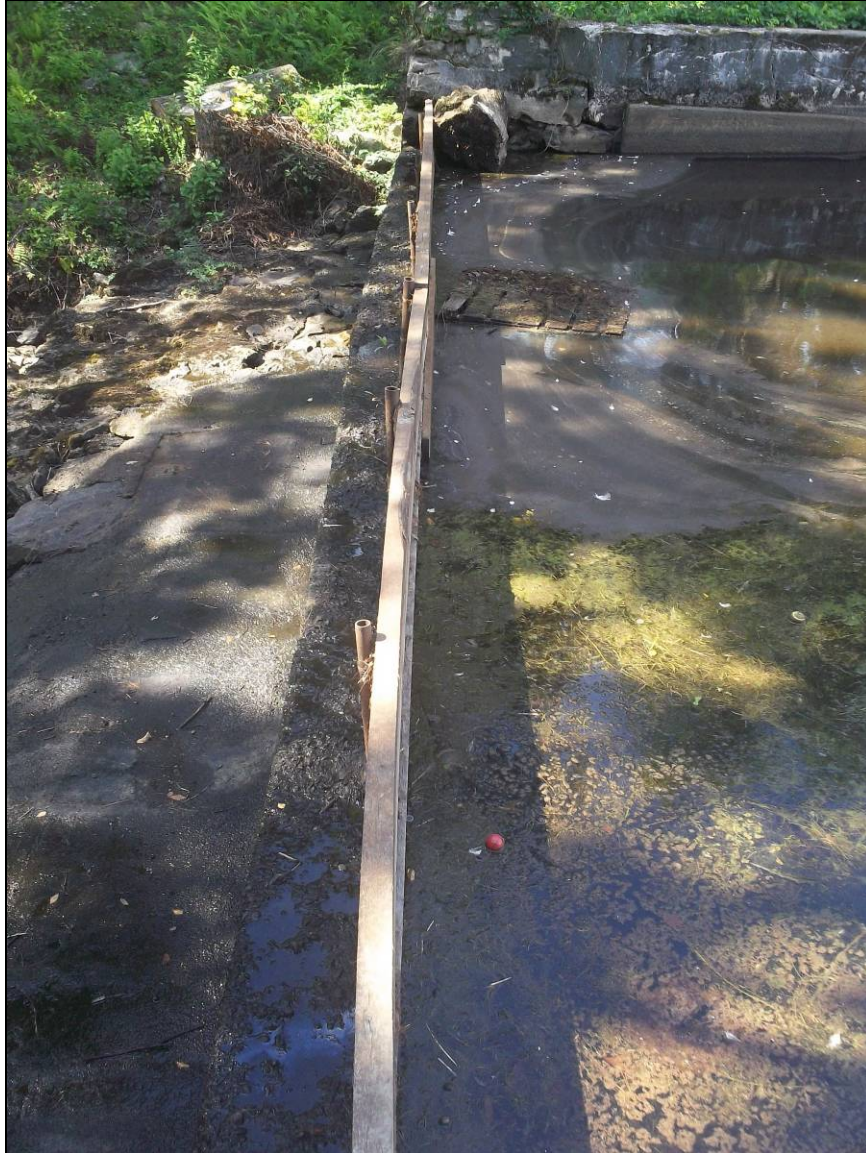
Photo 13: Overview of weir
