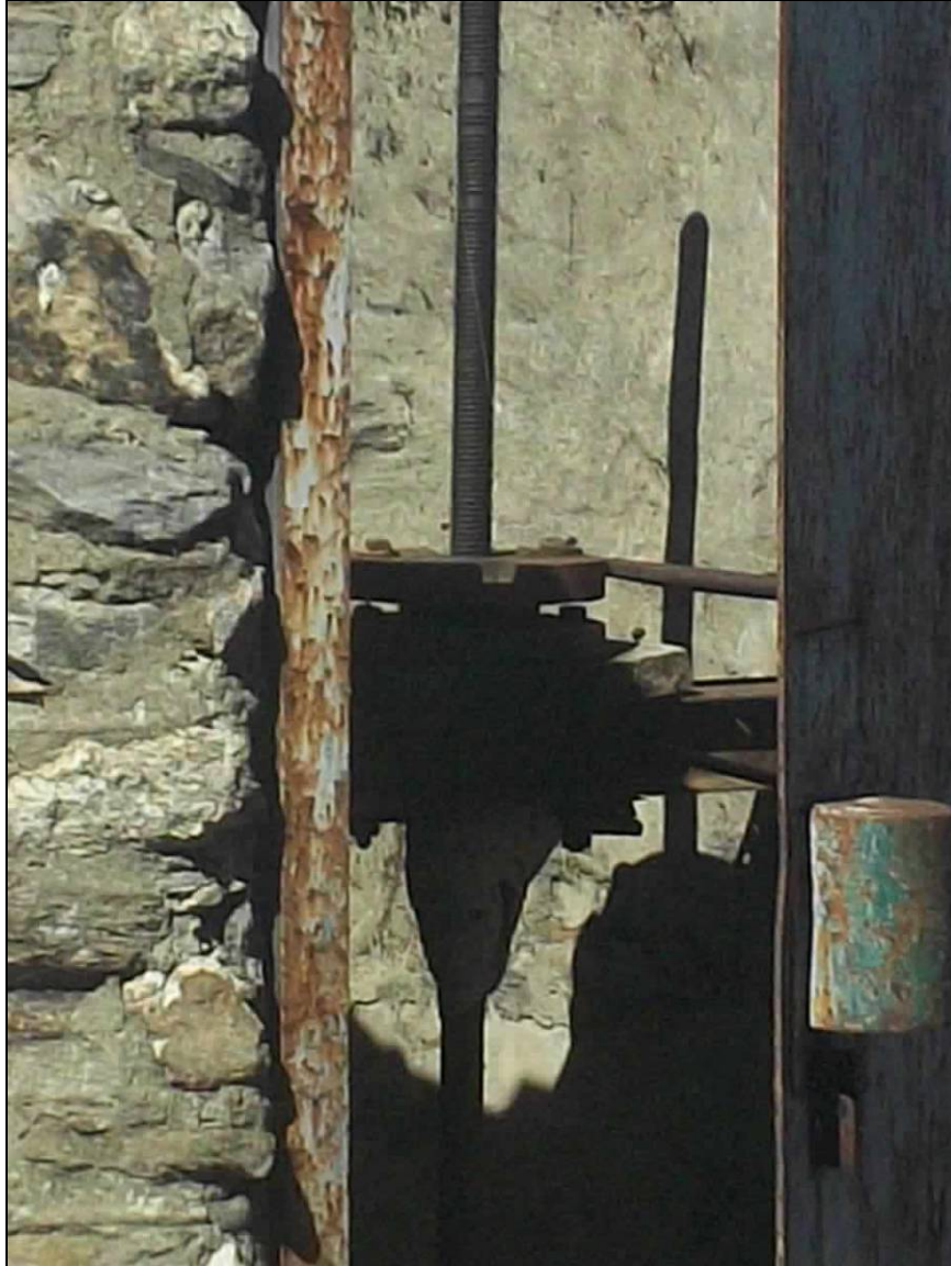
Photo 17: Overview of gatehouse interior & operator
