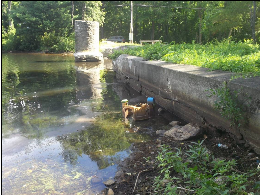
Photo 3: Overview of upstream face from right abutment
