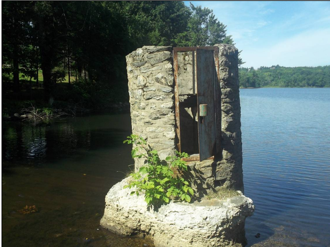
Photo 16: Overview of gatehouse exterior
