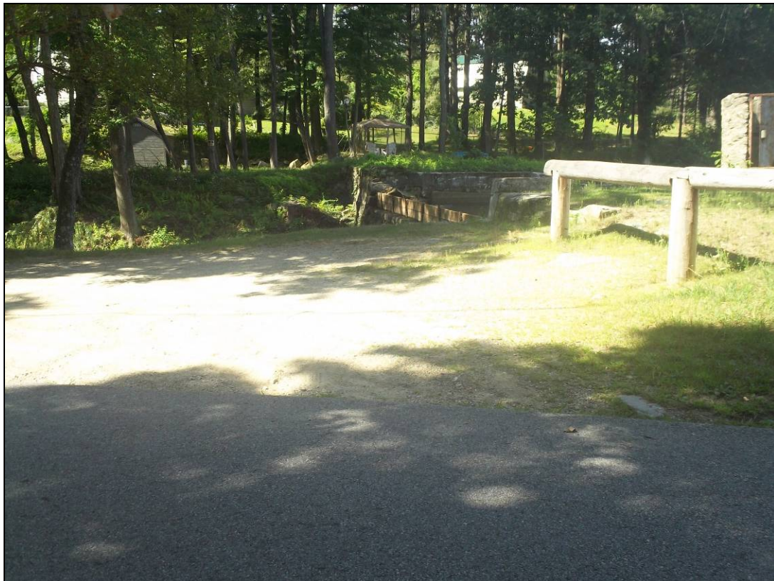
Photo 8: Overview of downstream face from left abutment
