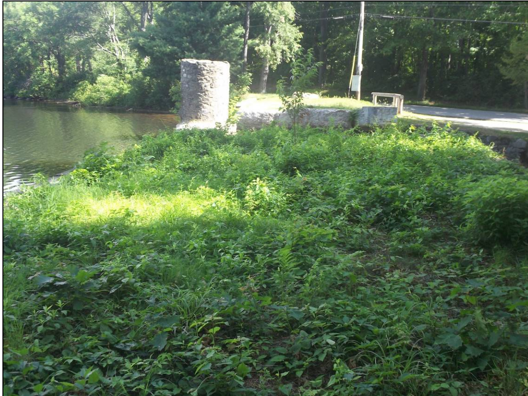
Photo 5: Overview of dam crest from right abutment
