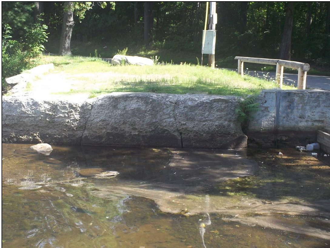
Photo 12: Overview of left training wall
