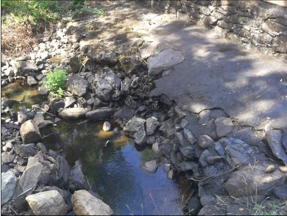
Photo 14: Overview of stilling basin
