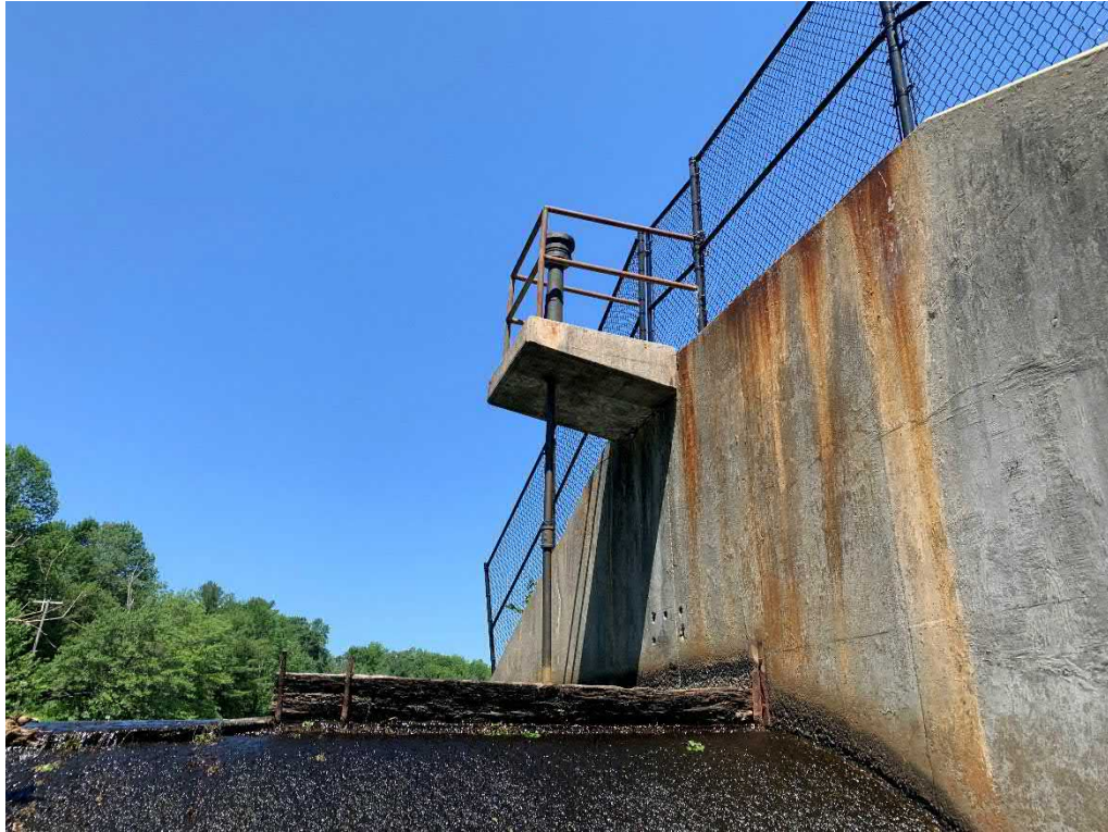
Photo 15: Overview of gatehouse exterior – note new chain link fence
