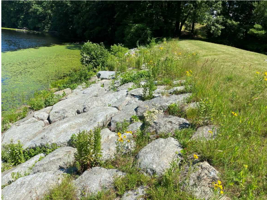
Photo 3: Overview of upstream face from right abutment
