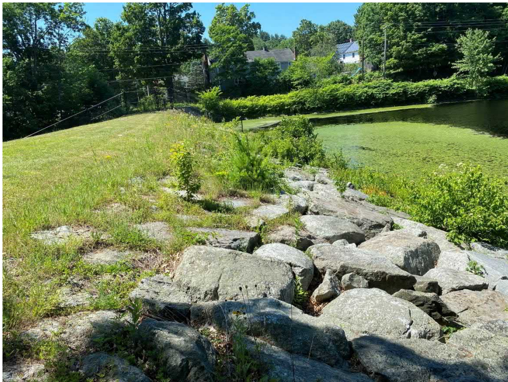
Photo 4: Overview of upstream face from left abutment
