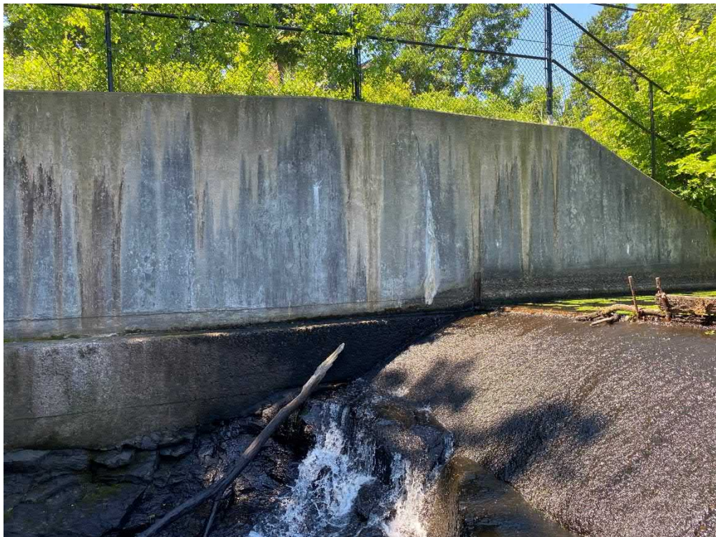
Photo 10: Overview of right training wall
