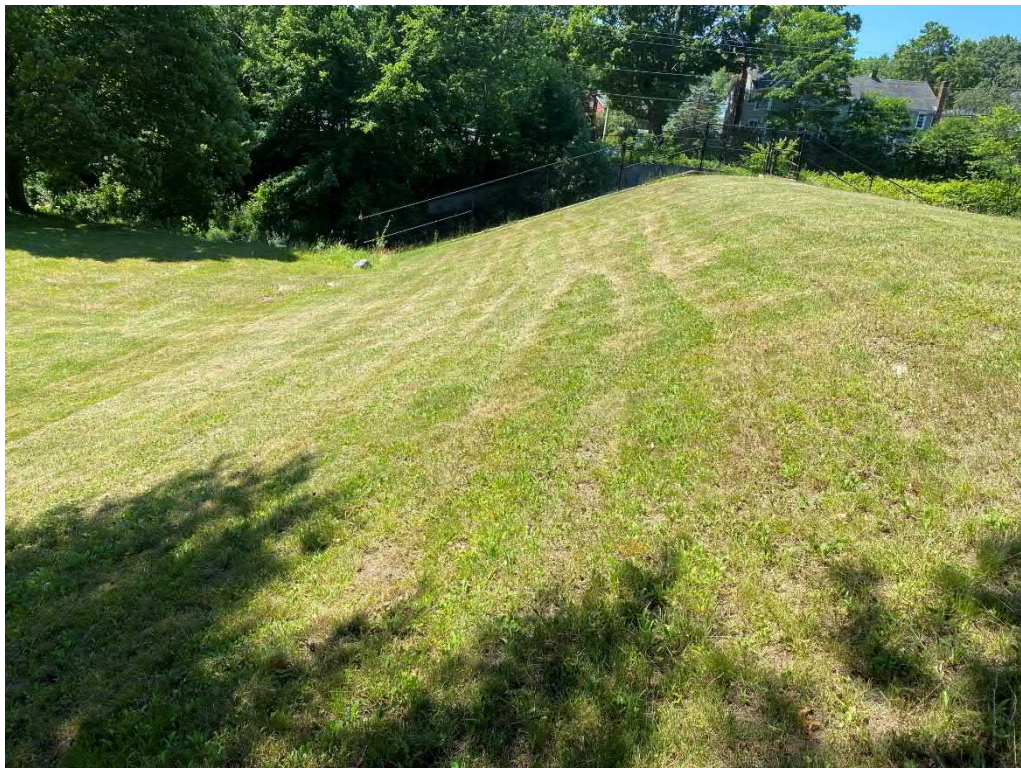
Photo 8: Overview of downstream face from left abutment
