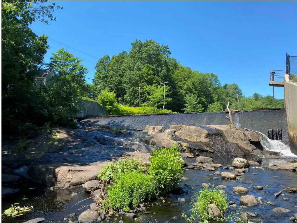
Photo 9: Overview of spillway from downstream (tailrace or channel area)
