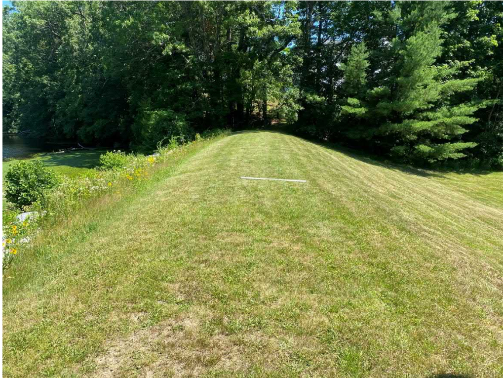
Photo 5: Overview of dam crest from right abutment
