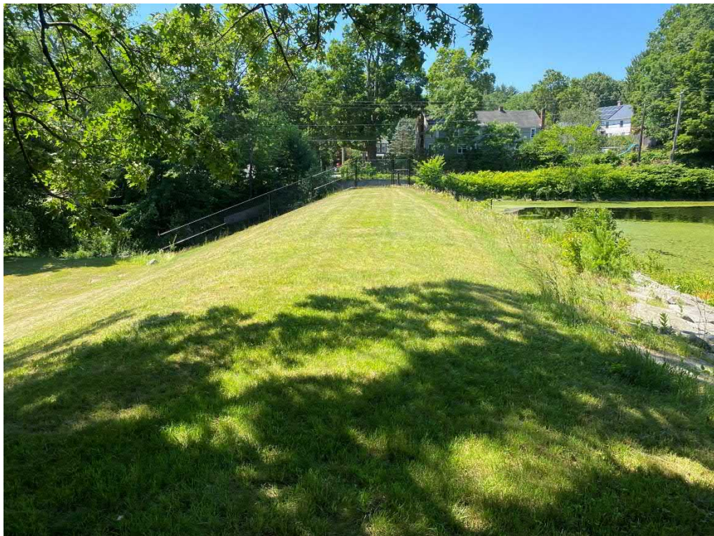
Photo 6: Overview of dam crest from left abutment
