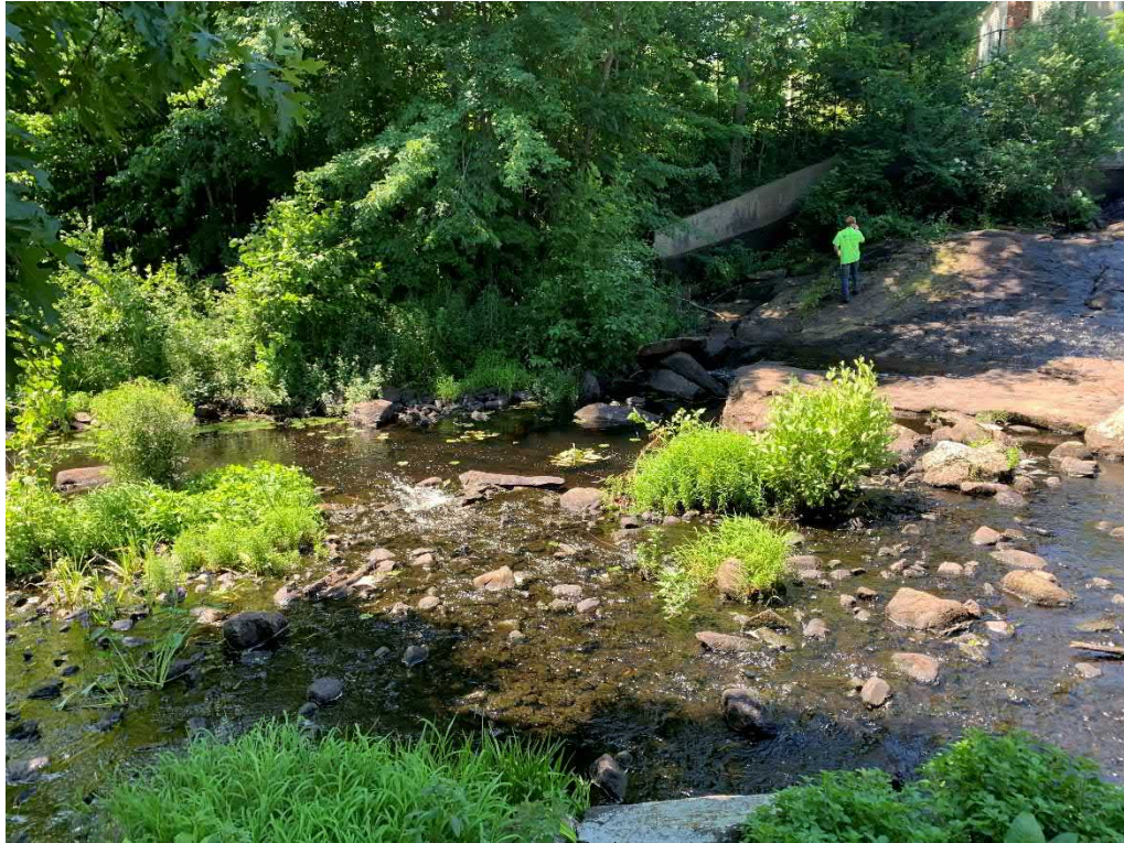
Photo 13: Overview of stilling basin
