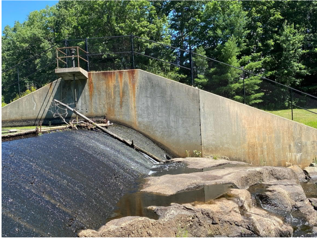
Photo 11: Overview of left training wall
