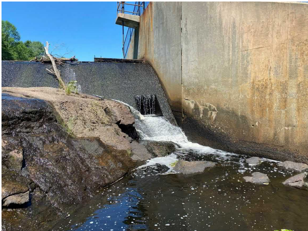
Photo 18: Low level outlet through spillway
