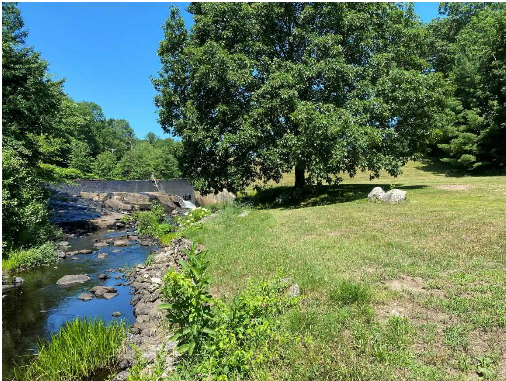
Photo 2: Overview of dam from downstream
