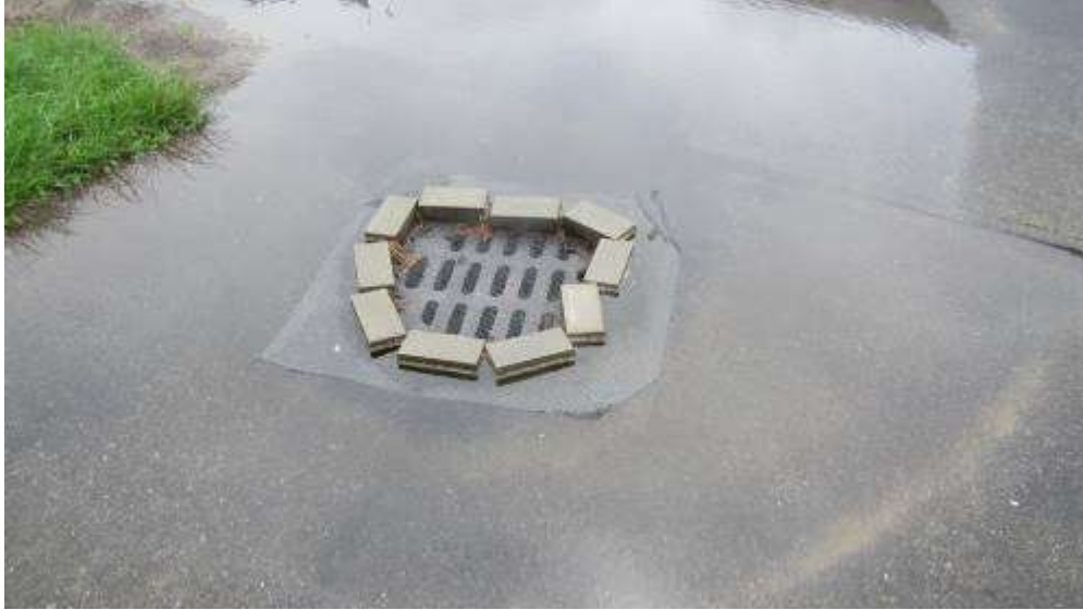
Brick dammed drain in courtyard
