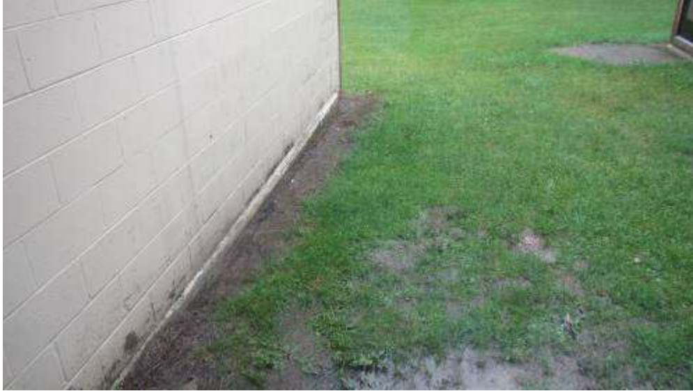
Example of flashing on other exterior walls of LMS
