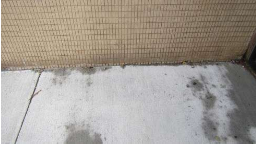
Exterior wall covering consisting of 1" x 2" ceramic tiles
