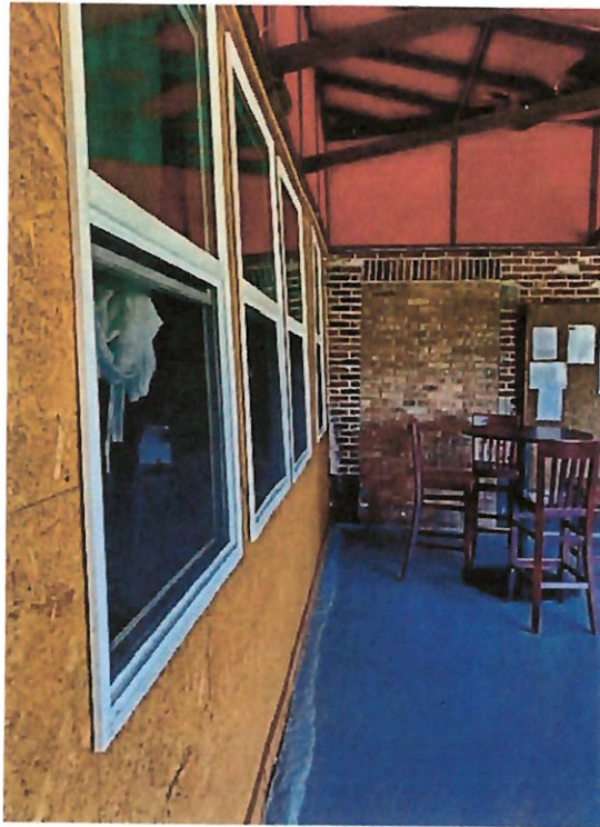
Photograph #15 – Exterior Bar Wall Lean
