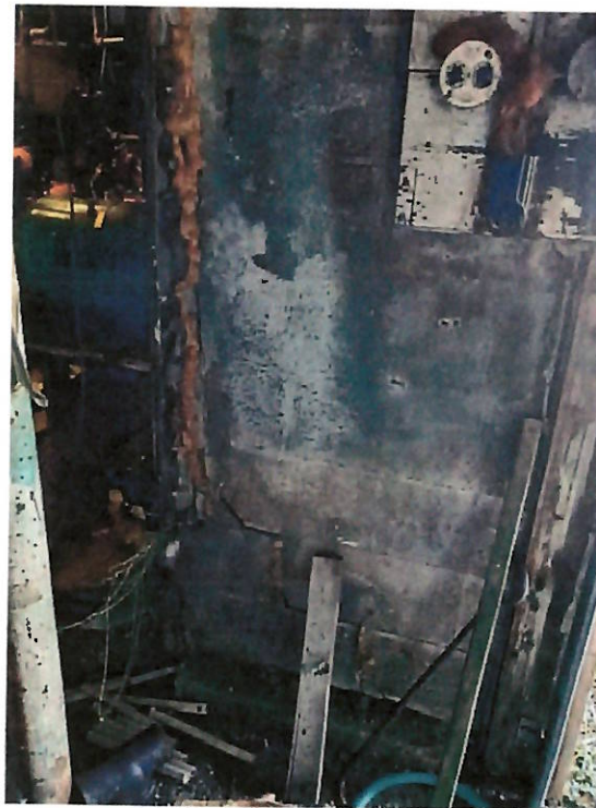
Photograph #4 – Cracked Foundation Wall
