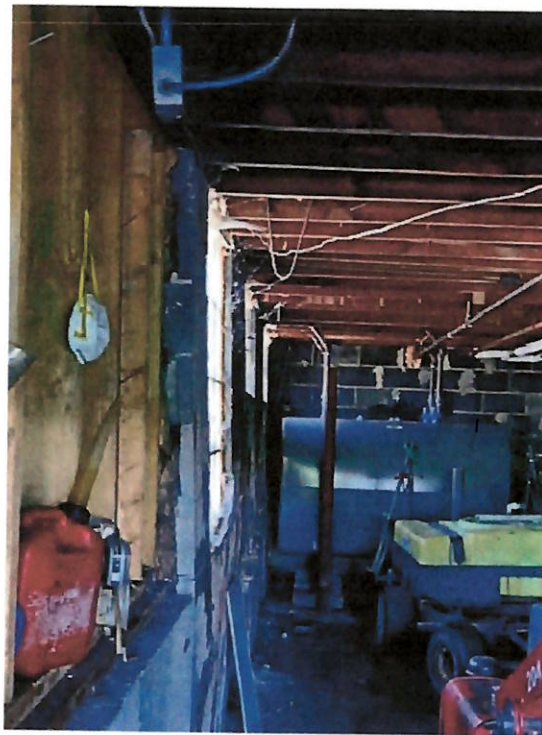
Photograph #2 – Leaning Foundation Wall
