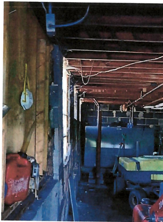
Photograph #2 – Leaning Foundation Wall
