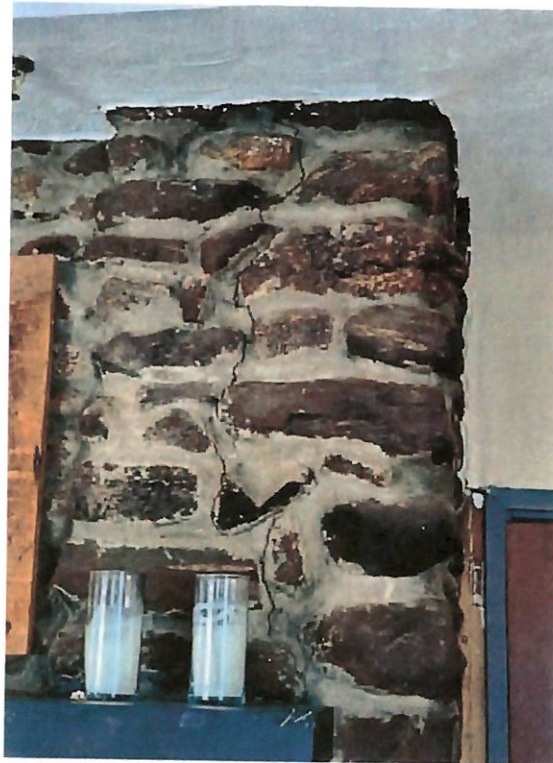
Photograph #19 – Cracked Stone Fireplace
