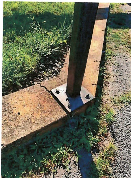
Photograph #12 – Cracked Foundation Wall
