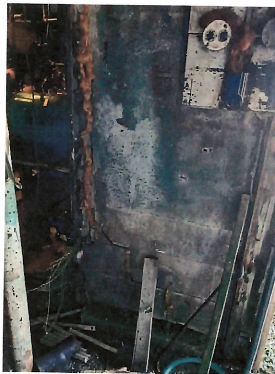
Photograph #4 – Cracked Foundation Wall
