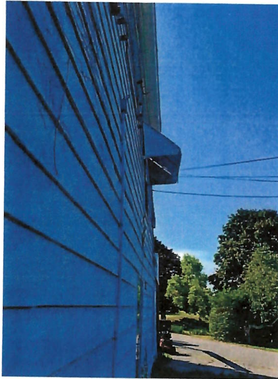
Photograph #1 – Bowed Exterior Wall
