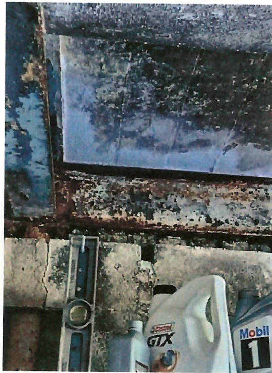
Photograph #21 – Corroded First Floor Beam
