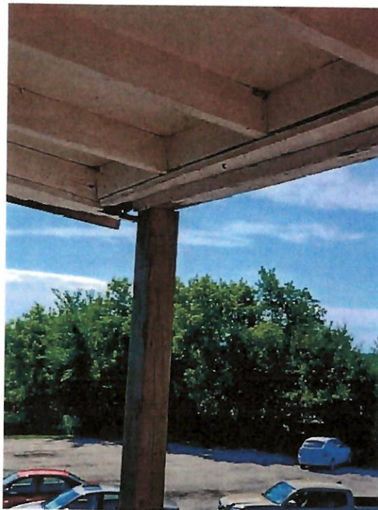
Photograph #14 - Deck Roof Beam Connection
