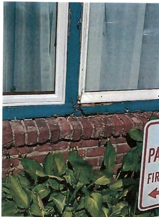
Photograph #28 – Rotted Window Frame
