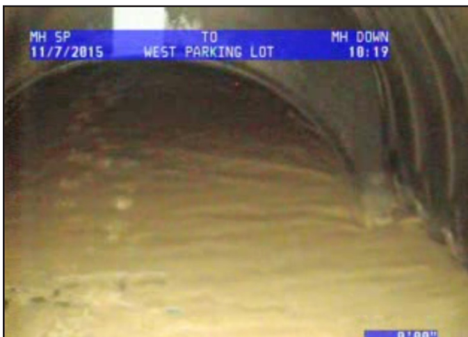
SEPARATOR ROW: Separator Row prior to cleaning
