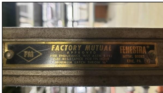
FIGURE 6: 90-MINUTE RATED FIRE DOOR
