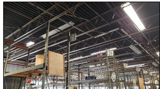
FIGURE 5: UNPROTECTED STEEL JOISTS (TYPE IIB CONSTRUCTION)
