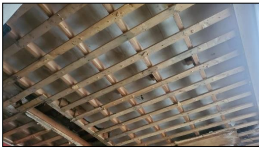
FIGURE 4: OFFICE WING COMBUSTIBLE FRAMING (TYPE VB CONSTRUCTION)
