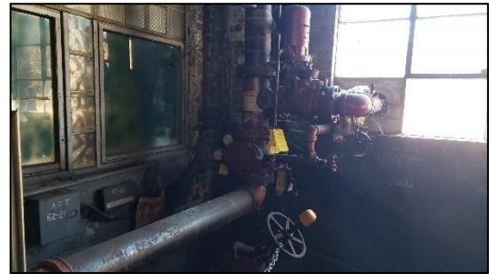
FIGURE 11: SPRINKLER ASSEMBLY (SPACE 3)
