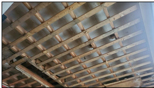
FIGURE 4: OFFICE WING COMBUSTIBLE FRAMING (TYPE VB CONSTRUCTION)
