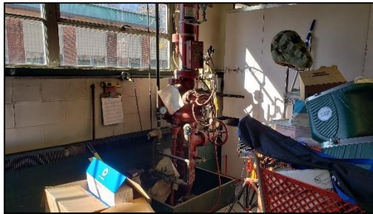
FIGURE 10: SPRINKLER ASSEMBLY (SPACE 10)
