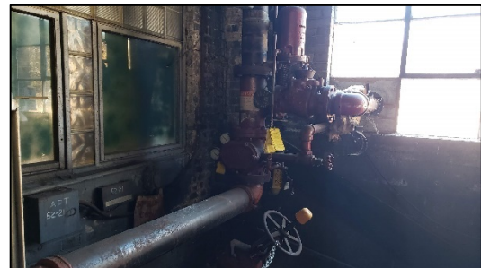
FIGURE 11: SPRINKLER ASSEMBLY (SPACE 3)
