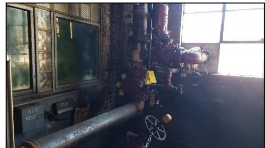
FIGURE 11: SPRINKLER ASSEMBLY (SPACE 3)
