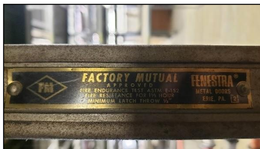
FIGURE 6: 90-MINUTE RATED FIRE DOOR
