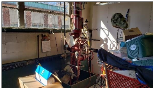
FIGURE 10: SPRINKLER ASSEMBLY (SPACE 10)
