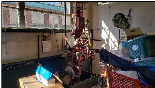
FIGURE 10: SPRINKLER ASSEMBLY (SPACE 10)
