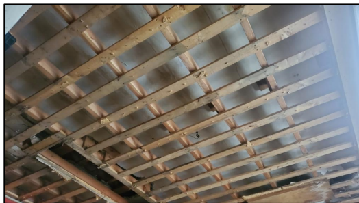
FIGURE 4: OFFICE WING COMBUSTIBLE FRAMING (TYPE VB CONSTRUCTION)
