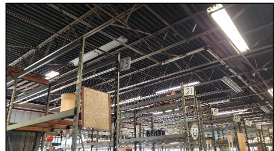
FIGURE 5: UNPROTECTED STEEL JOISTS (TYPE IIB CONSTRUCTION)
