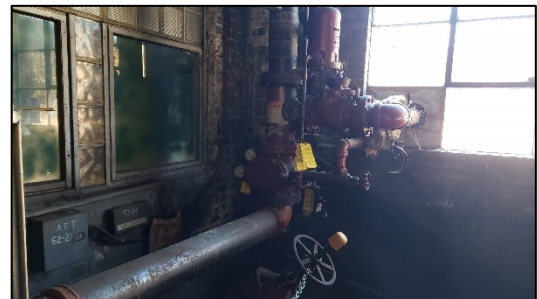
FIGURE 11: SPRINKLER ASSEMBLY (SPACE 3)
