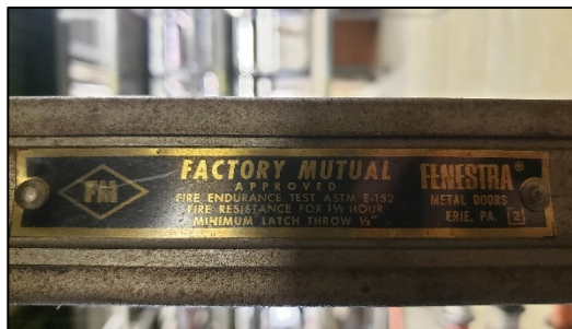
FIGURE 6: 90-MINUTE RATED FIRE DOOR
