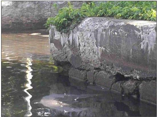
Photo 23: Areas of specific deficiencies-undermined cracked wall
