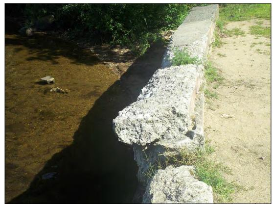
Photo 21: Areas of specific deficiencies-deteriorating concrete, leaning wall
