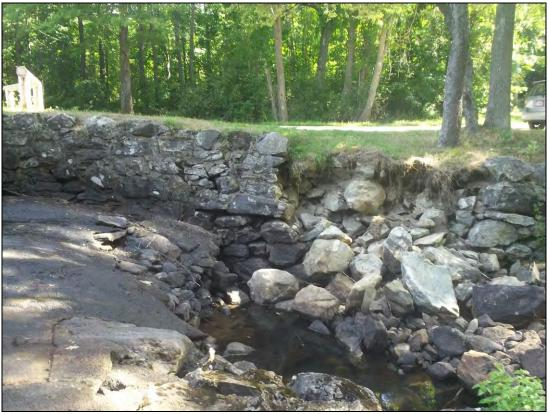
Photo 22: Areas of specific deficiencies-collapsed masonry wall
