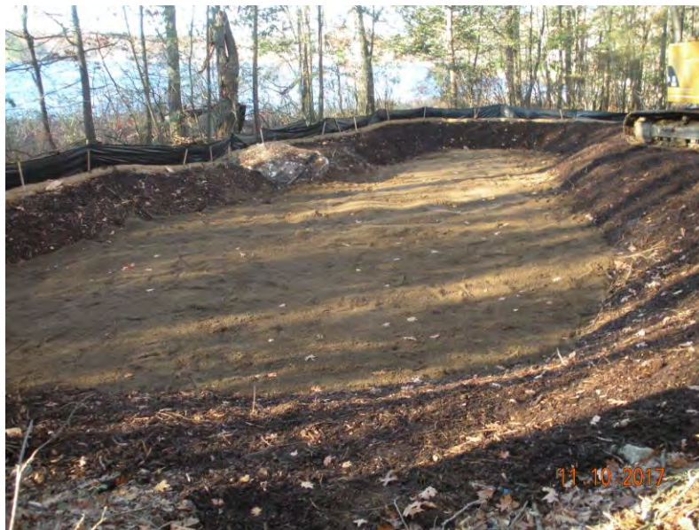
2. Finish graded and stabilized replication area
