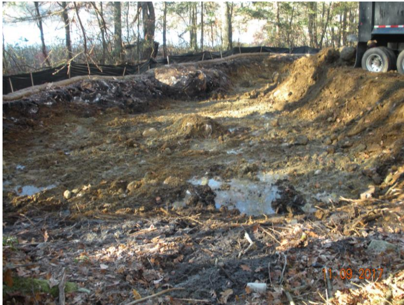
1. Replication area sub-grade with observed water table and redox features
