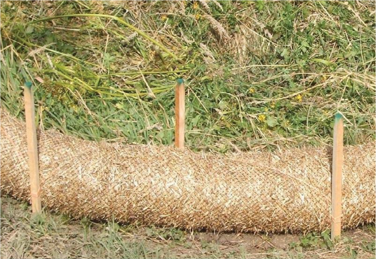
STRAW WATTLE – SHALLOW SLOPE ( \leq 4:1 ) (ALTERNATE STAKING)
