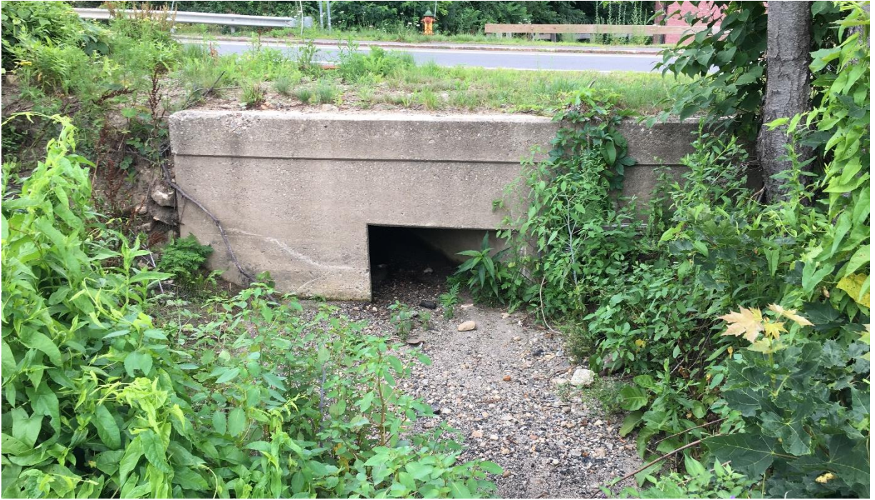
Photo #3: View of the culverted Grindstone Brook (intermittent stream) which flows under Main Street. The proposed duct bank will be installed over the culvert. Facing north.
