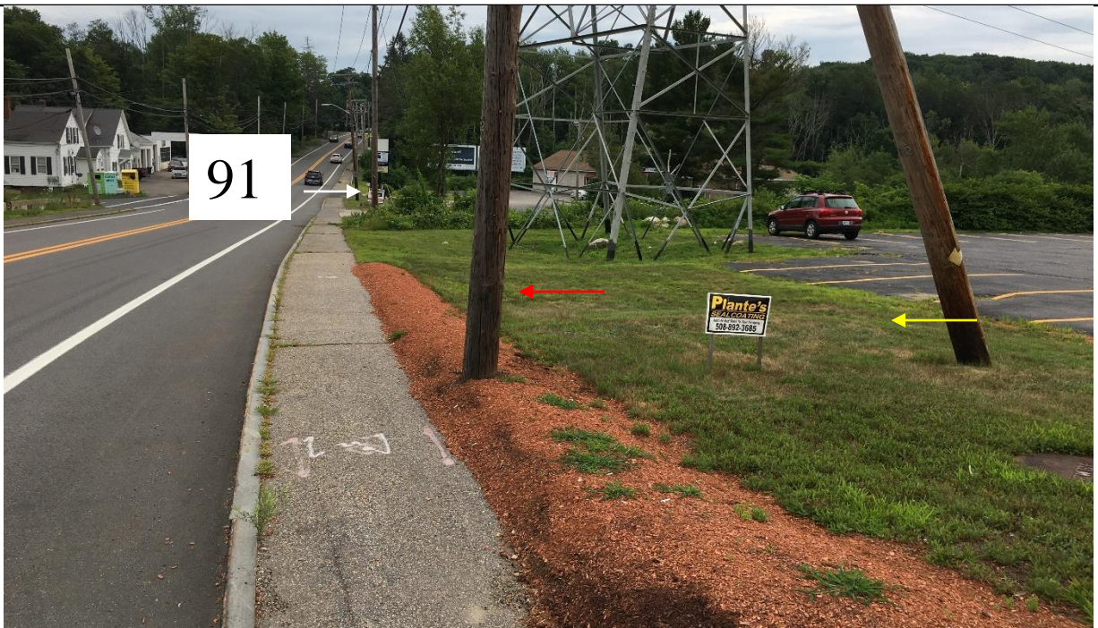
Photo #1: View along the existing distribution line along Main Street. UG conduit will be installed in the adjacent vegetated margin from Pole 92 (indicated by red arrow) to Pole 91 (indicated by white arrow) at which point the path will move within the sidewalk. Proposed pole P92-1 will be installed in the adjacent vegetated margin.(yellow arrow) Facing west.
