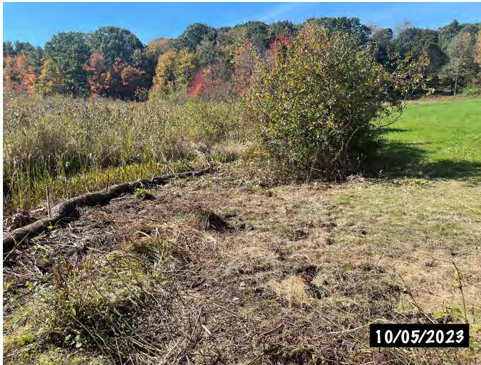
Picture 2. Looking west at the western end of the restoration area. Straw wattles can be seen on the left side, which acts as the limit of work and erosion/sedimentation control barrier, as required.
