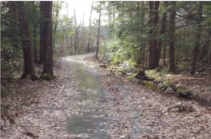
Photo 11. shows the paved roadway down to the pond. It is the route that the accessible pathway will follow. The cracked and raised pavement will be removed and additional gravel base will be laid down and a finish layer of ADA compliant stone grindings will be put down and compacted to provide the travel surface of the trail.
