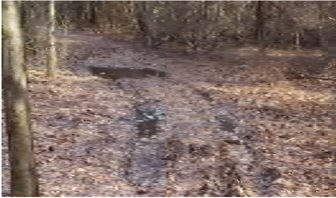
Photo 17. Shows standing water (mudpuddle) on the trail and the rutting caused when vehicles travel over this soft, wet soil. A technique called “turnpiking” will be used to resolve this issue by installing a bladder filled with trap rock and covering that with processed gravel.
