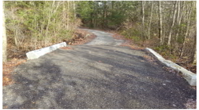
Photo 10. Depicts roadway at the stream crossing. The stream has been culverted under the roadway at this location. The new accessible trail will be a compacted ADA-compliant gravel surface that runs the entire length of the road from the parking area to the viewing platform.
