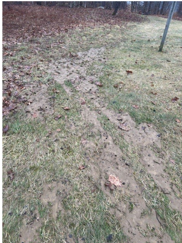
Photos 9-10. Pockets of sediment deposits observed within lawn and down gradient of the extension pipe discharge point.
