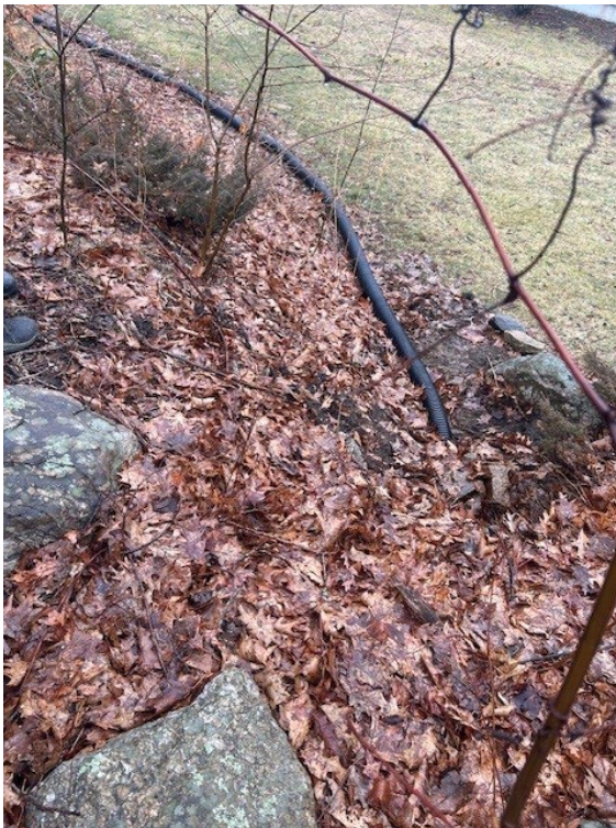
Photos 7 and 8. Stormwater culvert pipe extension at 525 Pine Street.
