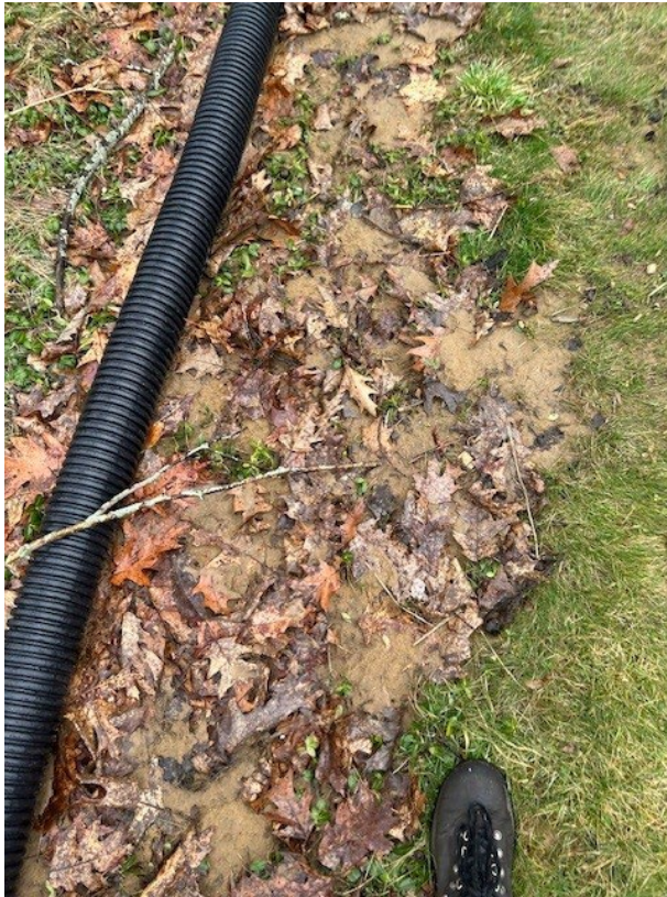
Photos 9-10. Pockets of sediment deposits observed within lawn and down gradient of the extension pipe discharge point.
