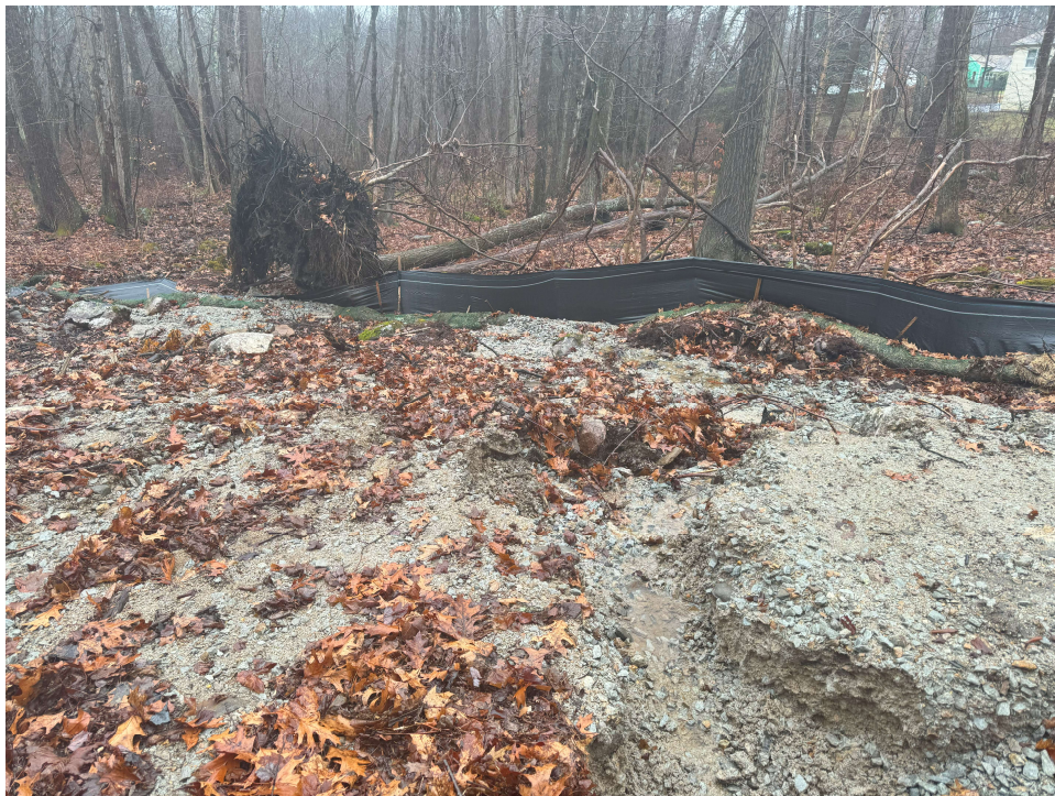
Photo 4 taken by EBT, Inc. on 12/28/2023 – Erosion gully discharging sediment into proposed replication area caused by recent storm event on 12/18/2023. The shown crushed stone was flushed into the proposed replication area (uplifted root system shown in photo is the same as in photo 3). The contractor filled the erosion gully, but in future storm events of similar size the stone will flush into the replication area again. A 6" minus rock lined shallow swale should be constructed to prevent erosion into the replication area in the future.
