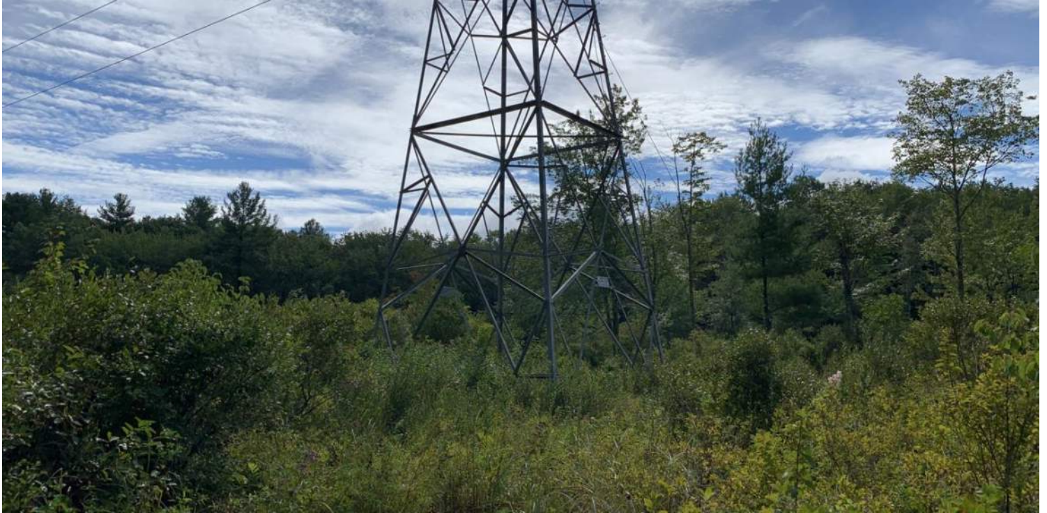
Photo #1: View of existing Structure 101 within BVW. Boring B-101 is proposed approximately 19 feet west of the existing structure within BVW. Temporary wetland matting will be used for the access and work pad related to this structure. Facing southeast
