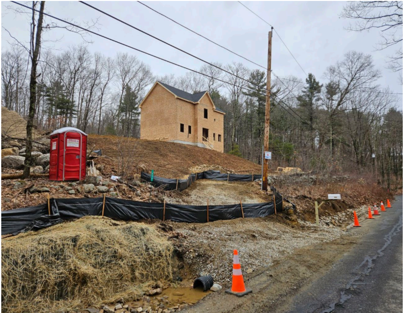
Photo 5. Photo provided by property owner of woodchips added to slope and haybale check dams added to driveway entrance on 3/6/2024.
