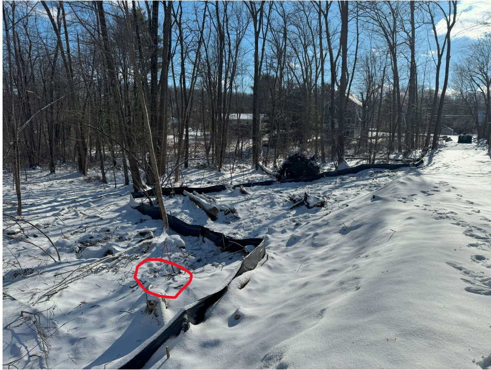
Photo 3 taken by EBT, Inc. on 1/17/2024 – Looking south showing replication area. Replaced pink WF 17 (WF 15 on the plan) is 6' outside of the erosion control barrier. On the plan it is at the limit of the replication area. The erosion control barrier should have been placed in the field exactly where shown on the plan – either the flag or silt fence is not where it is shown on the approved plan.
