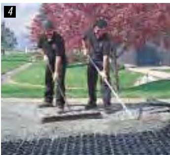
Fill rings with clean gravel.
