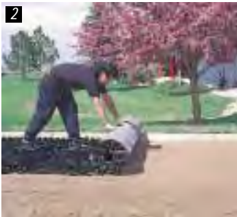
Roll out Gravelpave 2 , aligning the snap fit fasteners.
