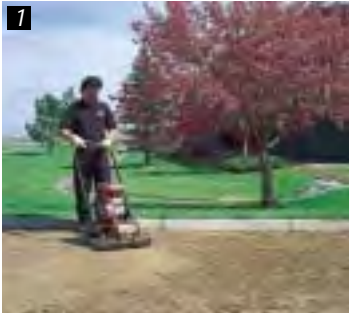
Place and compact sand and gravel base course.
