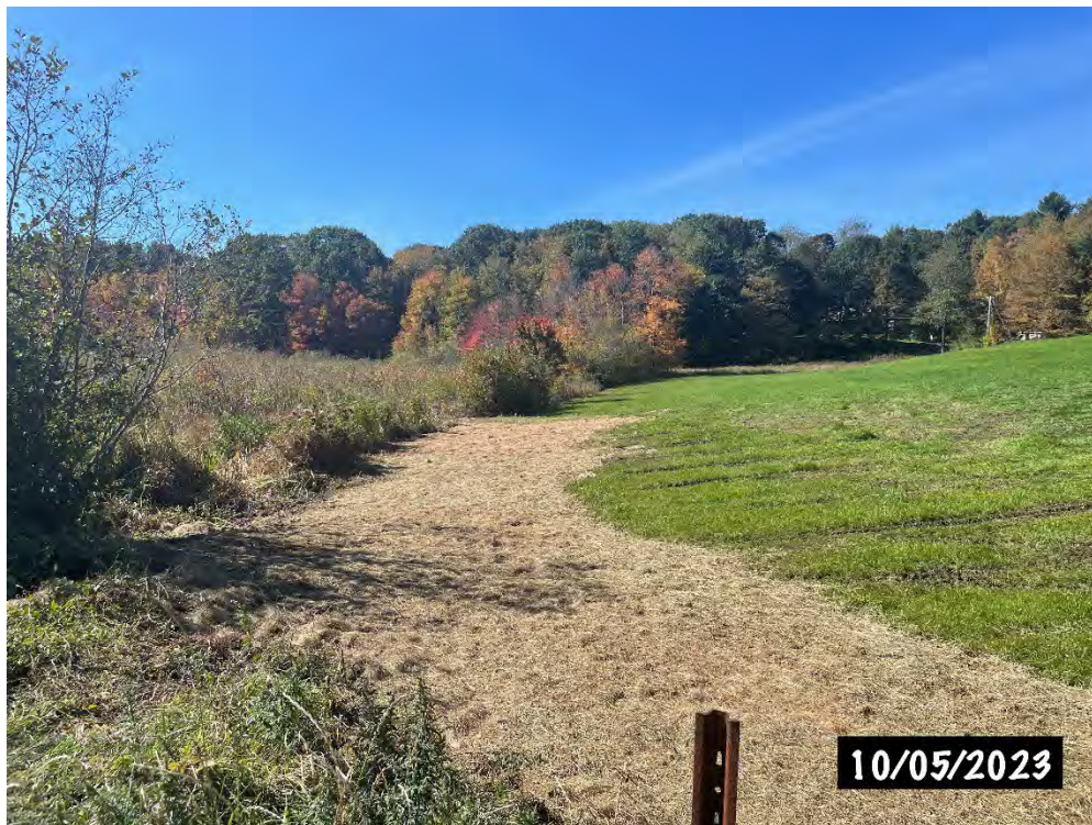
Picture 1. Looking west at the restored BVW from Watson Street. Straw was laid over the area of excavated spoil material as an erosion control practice.
