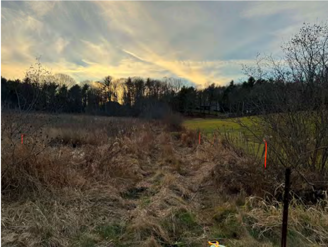
Photo 1 taken by EBT, Inc. on 11/25/2023 – Showing the 4 limit of fill flags and 2 depth of fill flags. The approximate volume of fill is 204.5 cubic yards.
