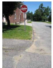
3. **Issue:** Sidewalk at the intersection of Market Street and Main Street has a cross slope >2%. Water is able to collect on surface of sidewalk.
