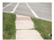
9. **Issue:** Crosswalk at intersection of route 9 and 56 does not have detectable warnings where pedestrian route crosses hazardous vehicular area.
