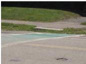
6. **Issue:** Curb ramp on Paxton street near town hall has a cracked and uneven surface. Transition at top and bottom of ramp is abrupt. There is no level landing at the top of the ramp.
