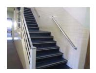
5. **Issue:** Stair handrails are not continuous. Handrails do not extend 12" at top and bottom of stairs. Tread nosings are abrupt.
